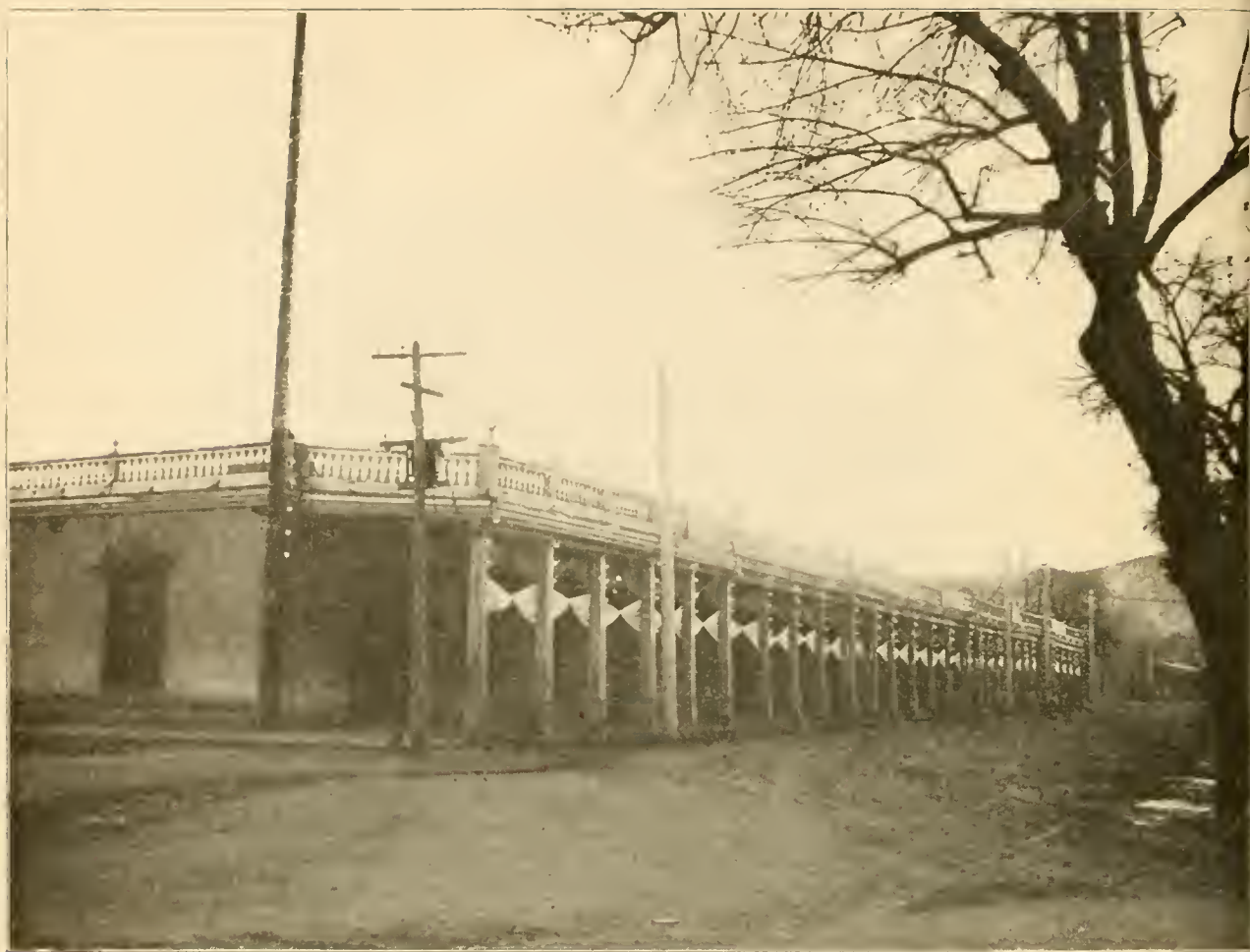
The Palace of the Governors as it Appeared on the Day of the Inauguration of the First State Governor January 15, 1912.
