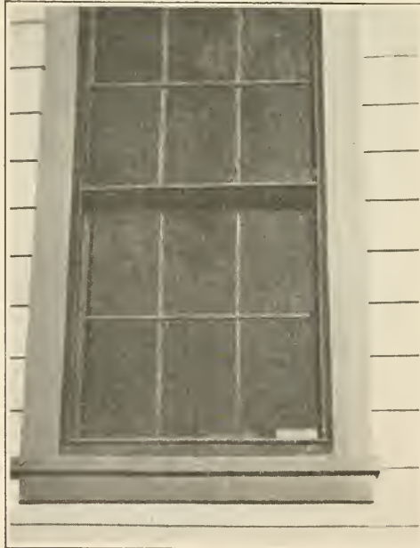
FIG. 141.—Close-up view of a window screen. This screen hangs from the top and is drawn up tightly against the battens on the sides and the sill on the bottom by a hook fitting in a ring attached to the inside of the sill.
