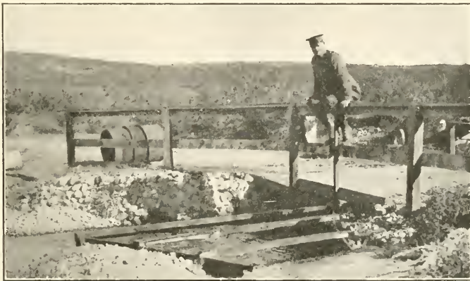
FIG. 114.—Utilizing a drip-can for a flowing stream. Note the drip-can fastened to the rail to the left of the officer.
