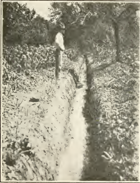
FIG. 65.—A common type of anti-mosquito ditch.
