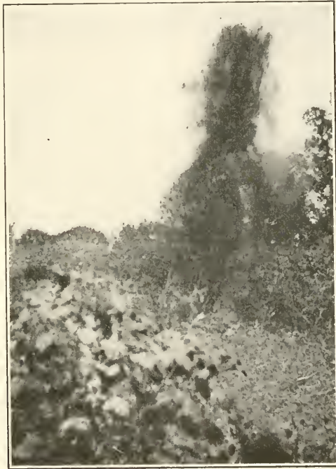
FIG. 75.—Blasting ditch in tangled underbrush.
