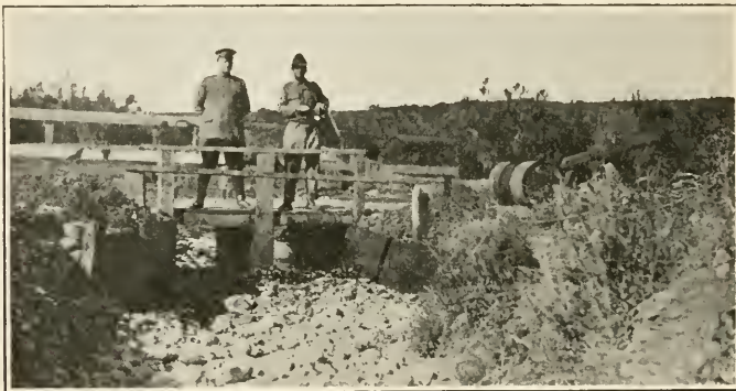
FIG. 52.—A culvert properly placed; it is neither too low nor too high. No pool can form about it.
