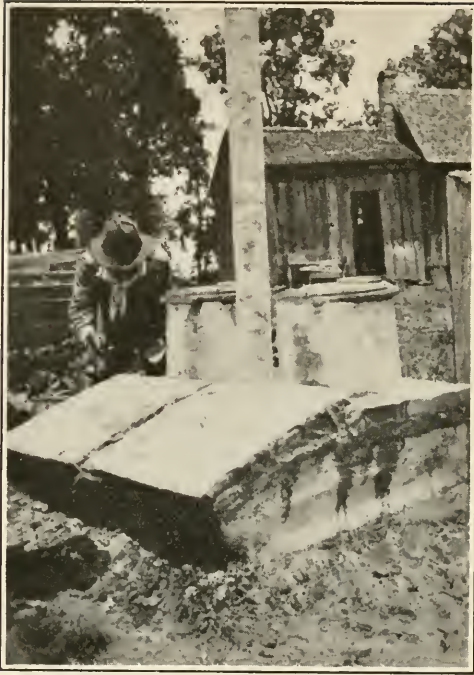
FIG. 145.—Making a concrete privy-vault mosquito-proof. All cracks are plastered over.
