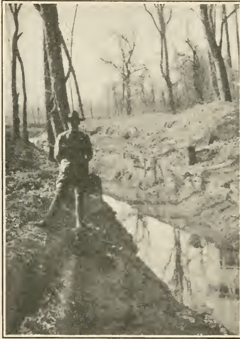
FIG. 97.—A new channel for a stream. Note the straight course and clean edges.
