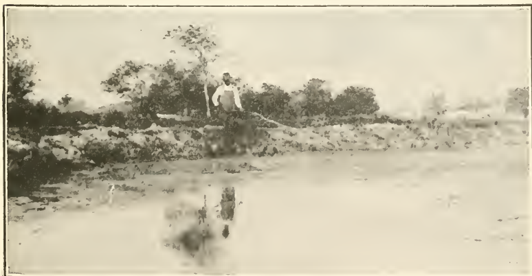
FIG. 133.—Treating pond with copper sulphate to kill algae. Laborer is dragging a small bag of the chemical through the water by means of a pole.
