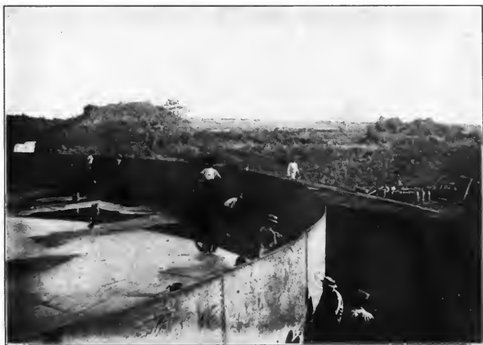
FIRST TANK ON ATLANTIC SIDE IN COURSE OF CONSTRUCTION.
