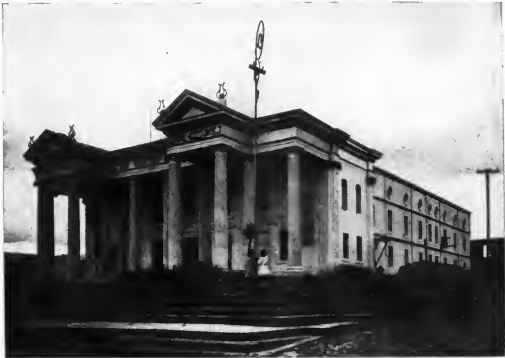
MUNICIPAL THEATER, QUEZALTENANGO, GUATEMALA.
