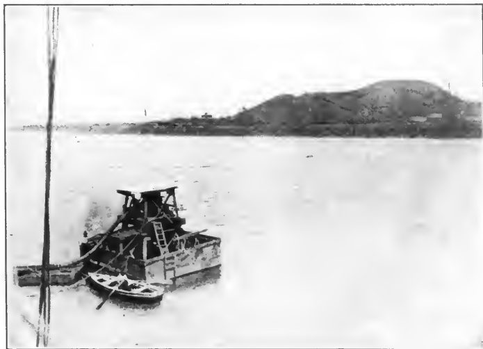
THE CRIB ON THE PACIFIC SIDE SEEN FROM THE TANK SHIP AND SHOWING THE HOSE THROUGH WHICH THE OIL IS PUMPED INTO THE SUBMERGED PIPE AND THEN ASHORE TO THE TANKS SEEN IN THE DISTANCE.
