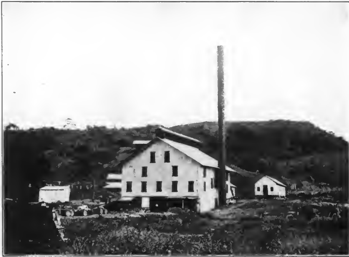
BOILER HOUSES, PACIFIC TERMINAL.
