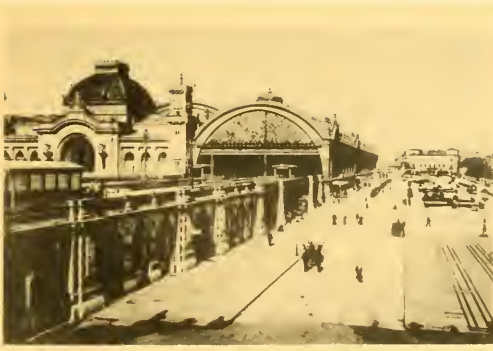
LXXVI. DRESDEN. VIADUCT AND RAILWAY STATION (HAUPT BAHN-HOF) PASSING ABOVE THE NORMAL STREET LEVEL, ILLUSTRATING THE TYPE PROPOSED IN THE OVERHEAD SCHEME FOR RAILWAY STATIONS WEST OF THE RIVER.
