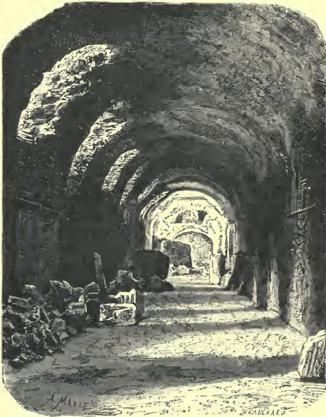
VAULTED PASSAGE BETWEEN THE PALACE OF TIBERIUS AND THE PUBLIC PALACE.
