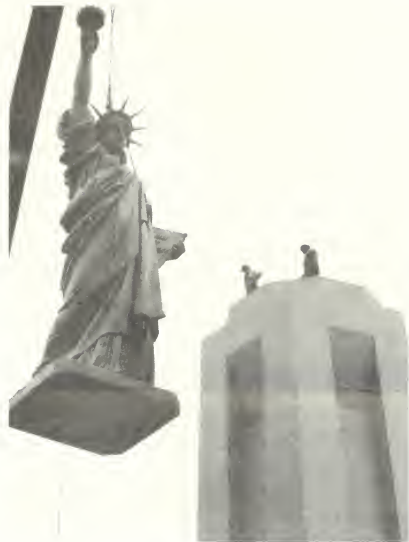
Installation of statue in Liberty Park
