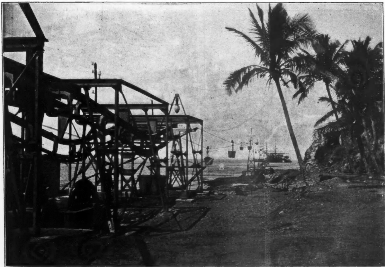
ROPEWAY FROM CENTRAL STATION TO LOADING BRIDGE
