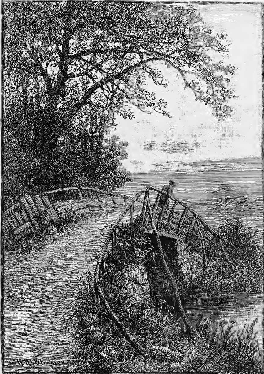
AN OLD BRIDGE.
