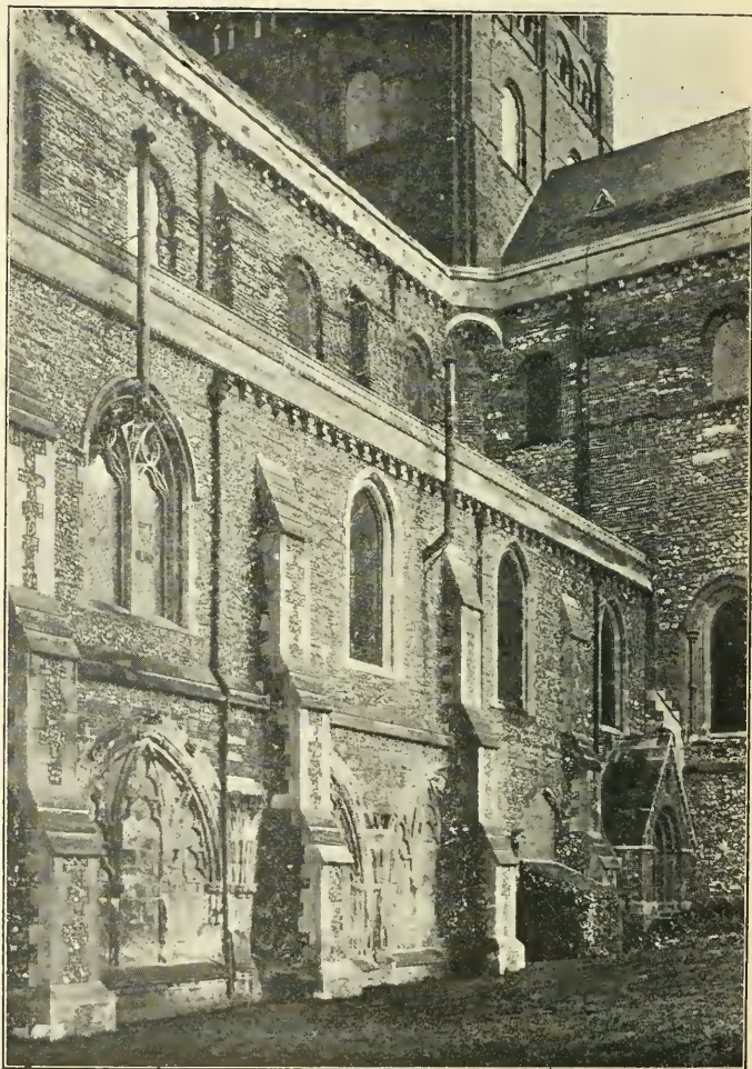
ANGLE BETWEEN NAVE AND TRANSEPT.
