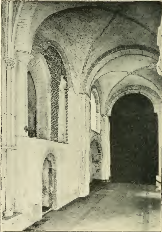
SOUTH AISLE OF PRESBYTERY.
