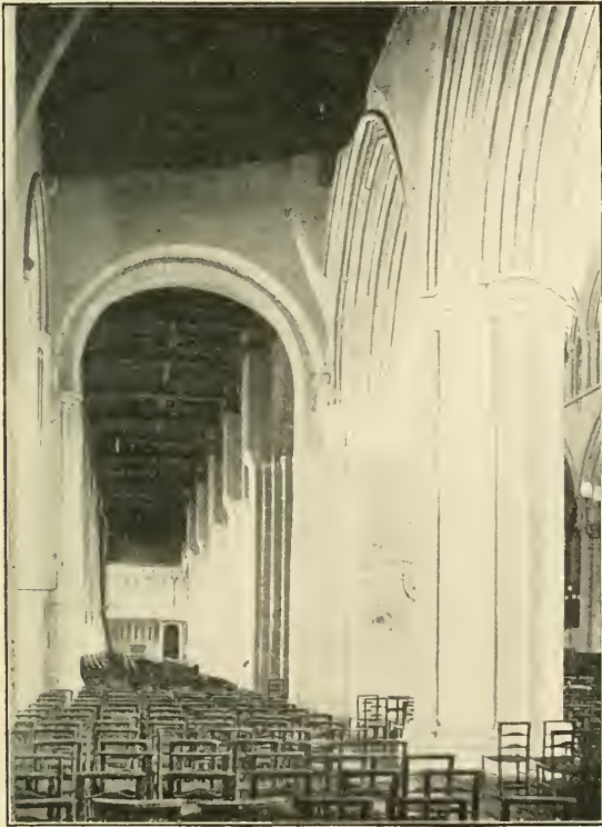
NORTH AISLE OF NAVE.
