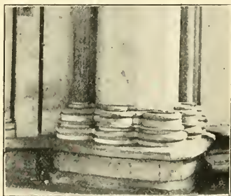
BASE OF INCOMPLETE PIER.
