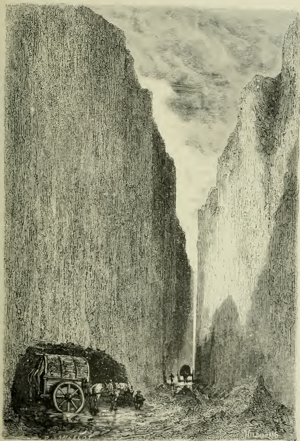
ROAD CUT THROUGH THE "YELLOW EARTH."
