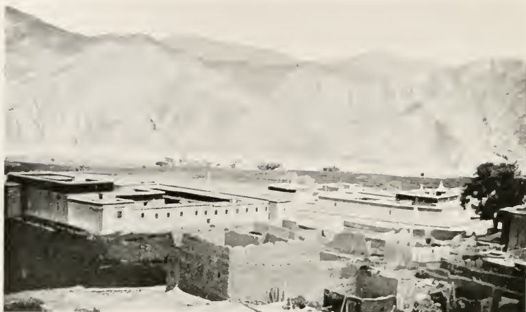
DRAYA JYAMDUN, LOOKING EAST
