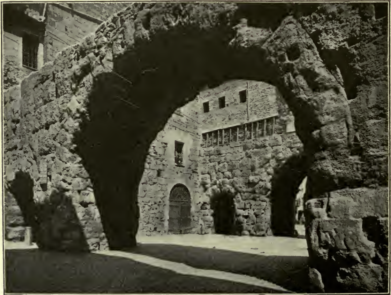
The gate by which the Pœnine Pass road left Aosta
