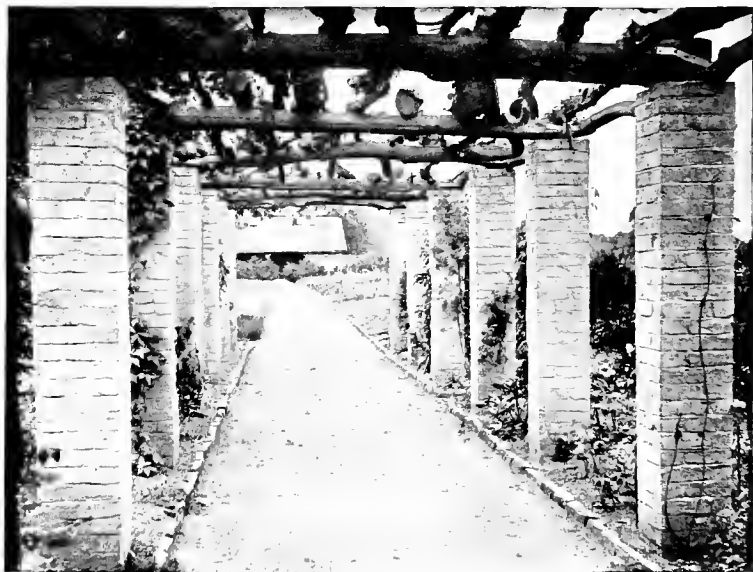
PERGOLA WITH BRICK PIERS AND BEAMS OF ROUGH OAK.
