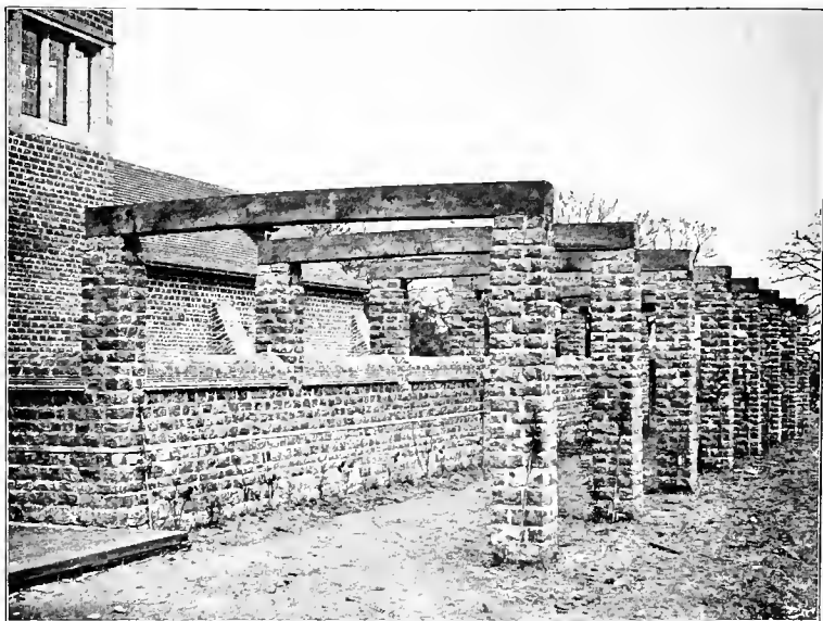
STONE-BUILT PERGOLA WITH WROUGHT OAK BEAMS.
