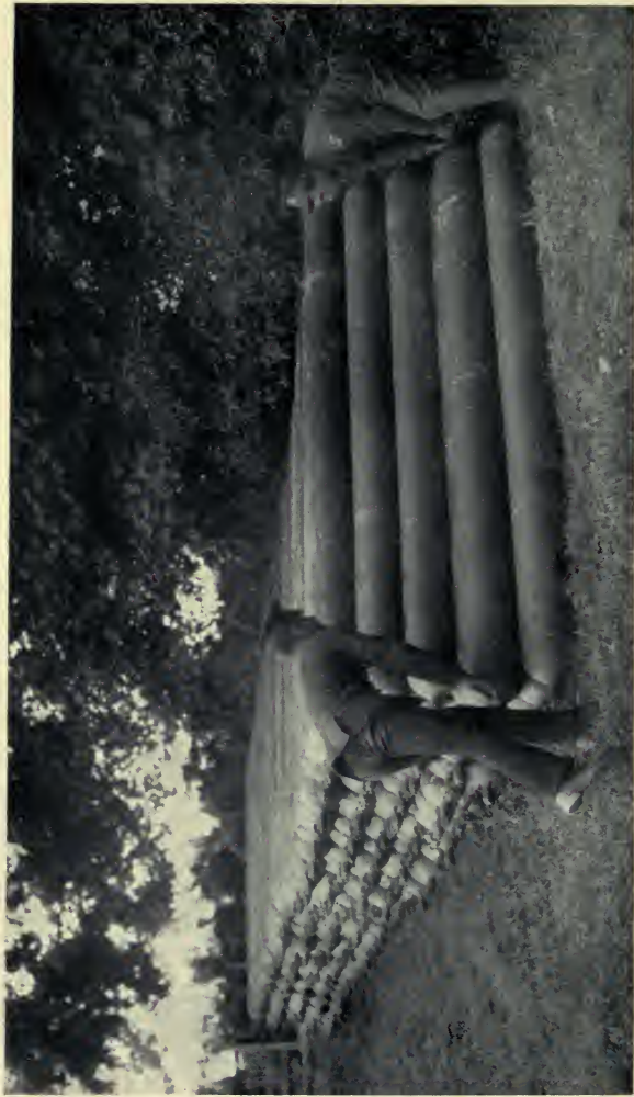
CYLINDERS OF HYDROGEN FOR INFLATING A BRITISH CAPTIVE MILITARY RECONNOITRING BALLOON.
