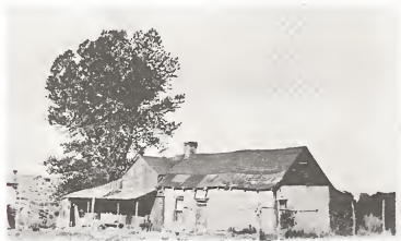
FIGURE 3-12 RANCH HOUSE LOCATED IN NYE COUNTY, 1927 SOURCE: NEVADA HISTORICAL SOCIETY, RENO, NEVADA
