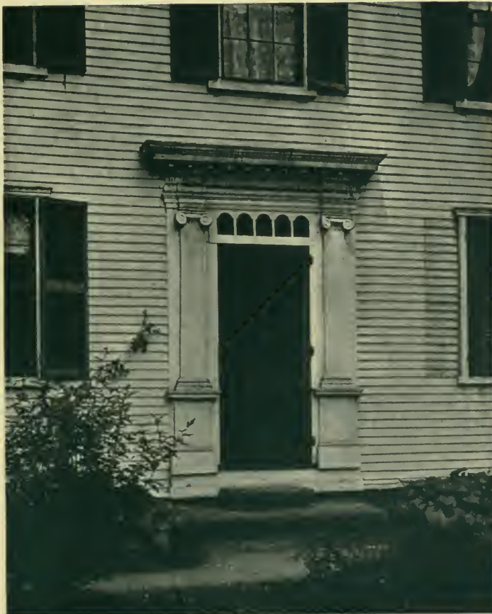
THE STEBBINS HOUSE, DEERFIELD, MASSACHUSETTS.
