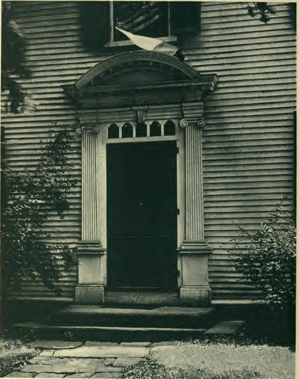
THE STEBBINS HOUSE, DEERFIELD, MASSACHUSETTS. Front Door Detail.
