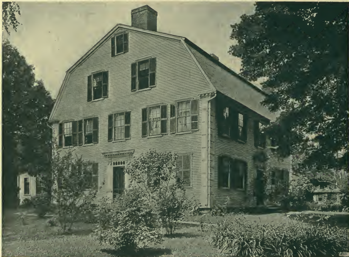
THE STEBBINS HOUSE, DEERFIELD, MASSACHUSETTS. Built about 1772.
