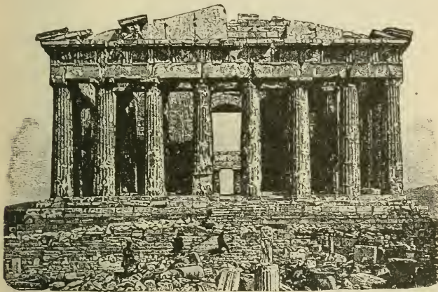
THE PARTHENON (present condition).
