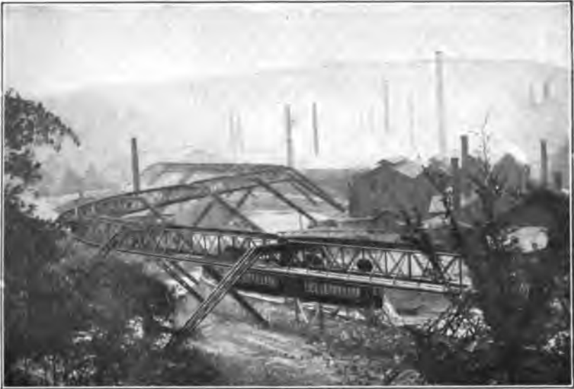
FIG. 1.—SUSPENDED RAILWAY AND TRAIN AT ELBERFELD.
