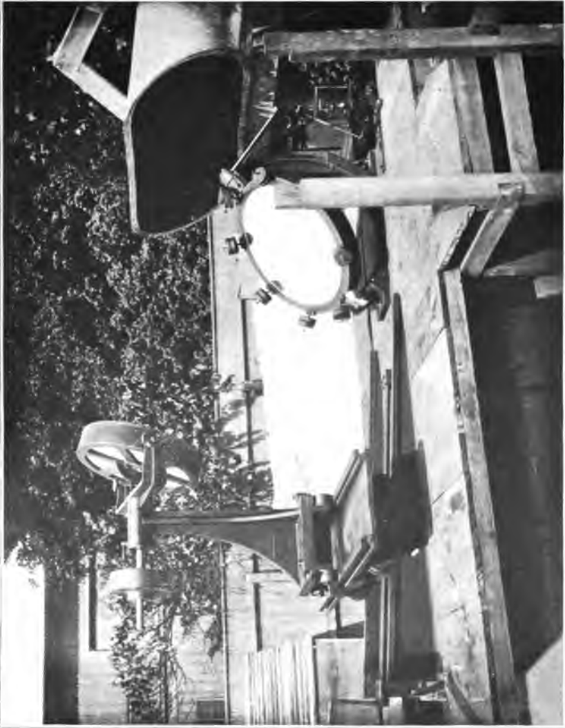
THE LARGE CŒLOSTAT WITH SECOND MIRROR, SMITHSONIAN ASTROPHYSICAL OBSERVATORY.
