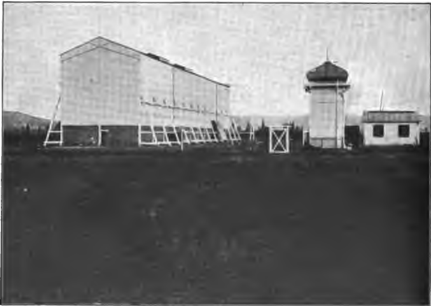
FIG. 2.—THE LEBAUDY SHED.
