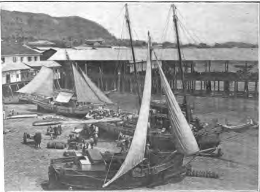
FIG. 2.—LOW TIDE IN THE HARBOR OF PANAMA. The range of tide at Panama is 20 feet, and at Colon only 1 foot.
