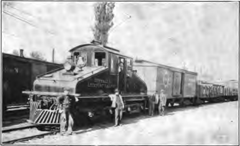
FIG. 1.—LOCOMOTIVE FOR THE BUFFALO AND LOCKPORT RAILWAY, GENERAL ELECTRIC COMPANY.
