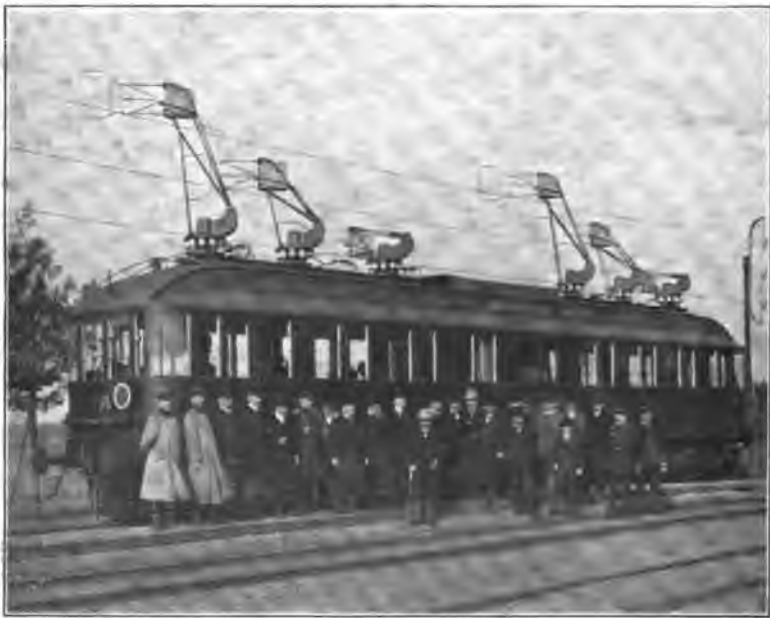
FIG. 2.—THE A. E. G. CAR USED IN THE MARIENFELDE-ZOSSEN HIGH-SPEED RUNS.
