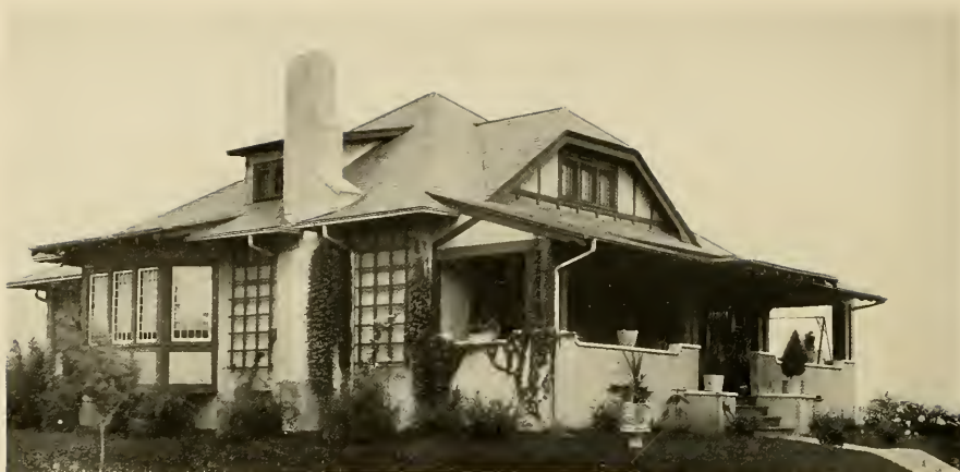
Atlas-White Semi-Bungalow Albany, N. Y.—D. Stuart Douglass, Architect
