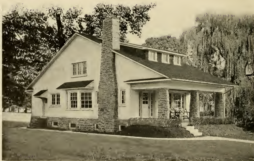
Stucco Bungalow, Narberth, Pa., Thomas Atherholt, Architect. Atlas-White Stucco over hollow tile.
