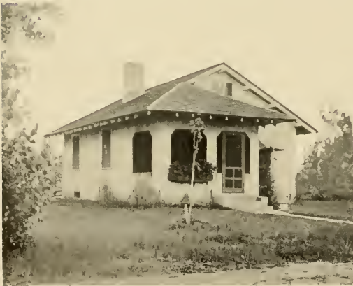
Bungalow of stucco over reinforced concrete. Milton Dana Morrill, Architect
