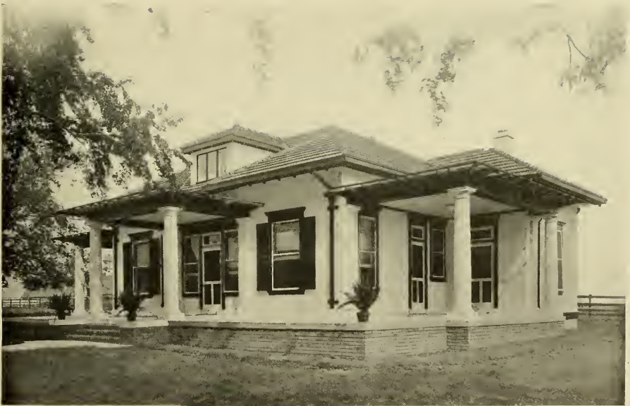
Atlas-White Stucco Bungalow, near Kansas City, Missouri. H. F. Hoit, Architect
