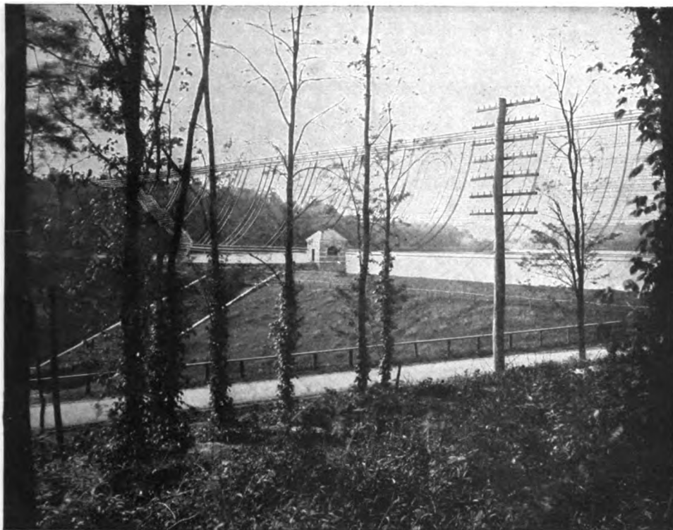
VIEW OF THE SPILLWAY AND DAM OF THE PRESENT KENSICO RESERVOIR
