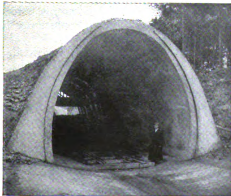
SECTION OF CUT-AND-COVER AQUEDUCT NEAR PEEKSKILL
