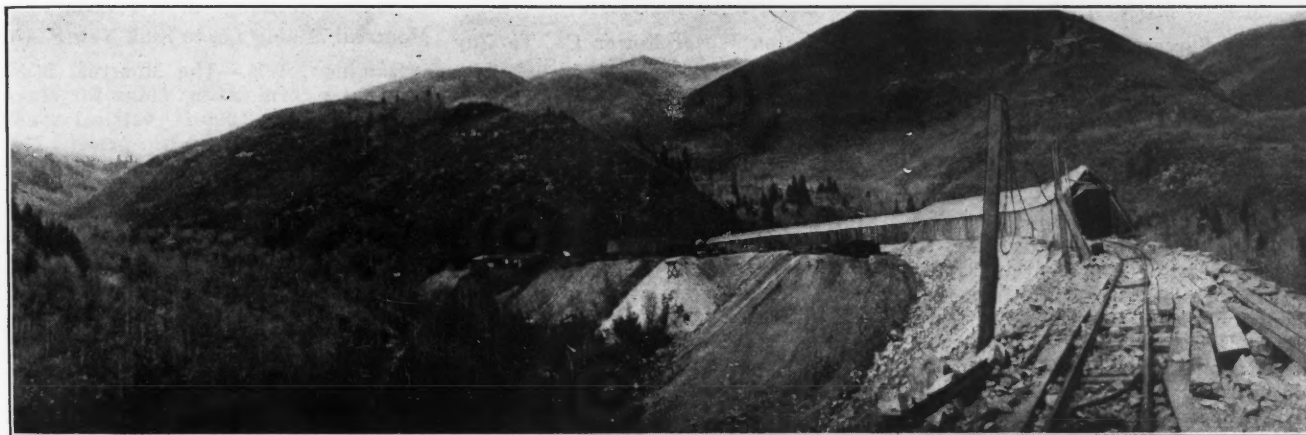
PORTAL AND SNOW SHEDS OF JUDGE MINING & SMELTING CO.'S SNAKE CREEK TUNNEL, LOOKING NORTHEAST TOWARD PARK CITY, UTAH
