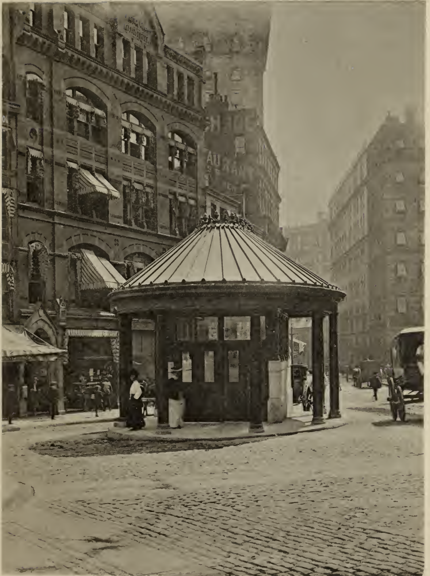
BUILDING OVER STAIRWAY TO EAST BOSTON TUNNEL IN COURT STREET NEAR SCOLLAY SQUARE, NEAR FORMER SITE OF WINTHROP STATUE. THE ROOF IS OF GLASS.
