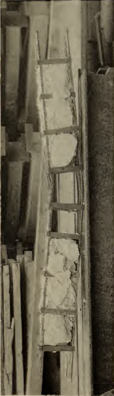
NO. 73 SHOWING STEEL SKELETON.
