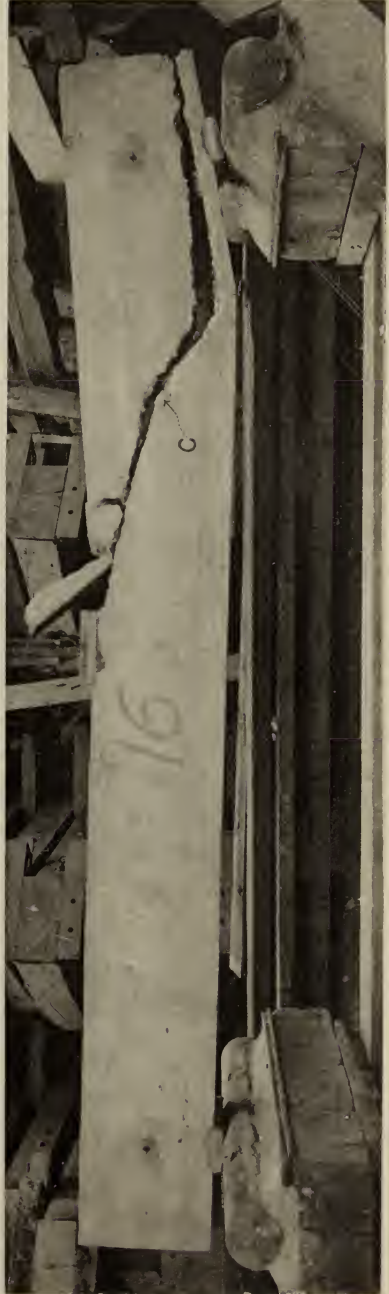
NO. 16 REINFORCED CONCRETE BEAMS.
