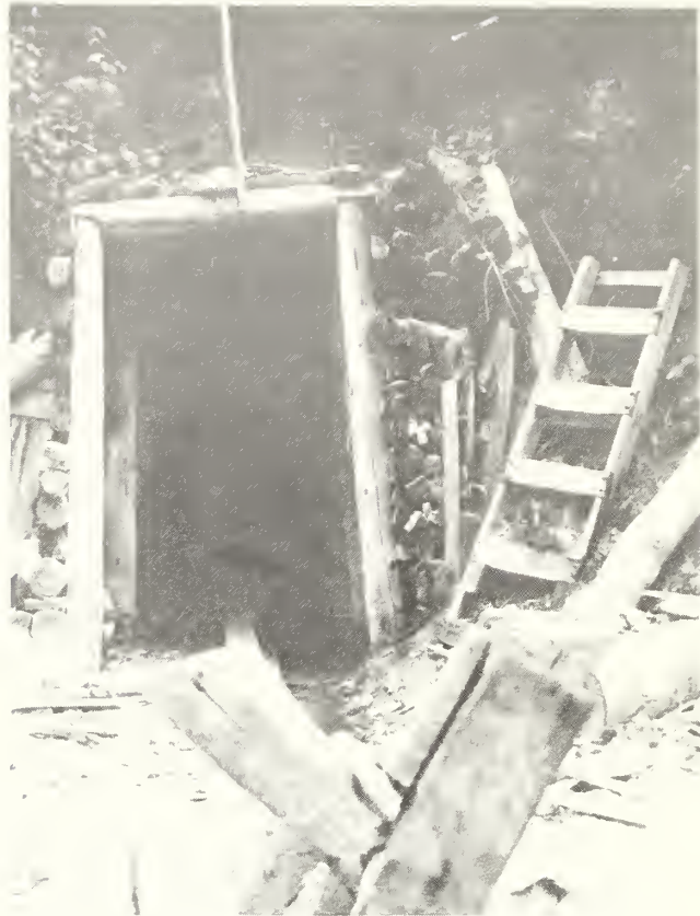
Test hole for the Cape Creek Tunnel.
