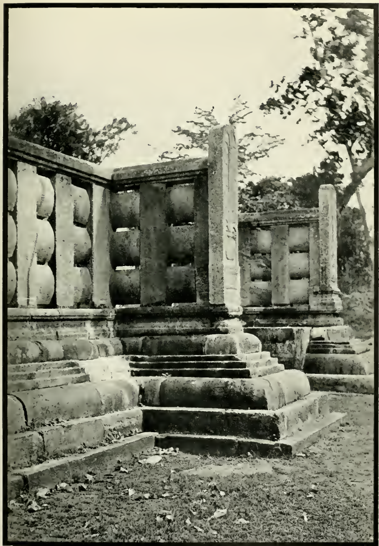
(RESTORED) STONE RAILING, AT ANURADHAPURA, BELONGING TO ABHAYAGIRIYA VIHARA.
