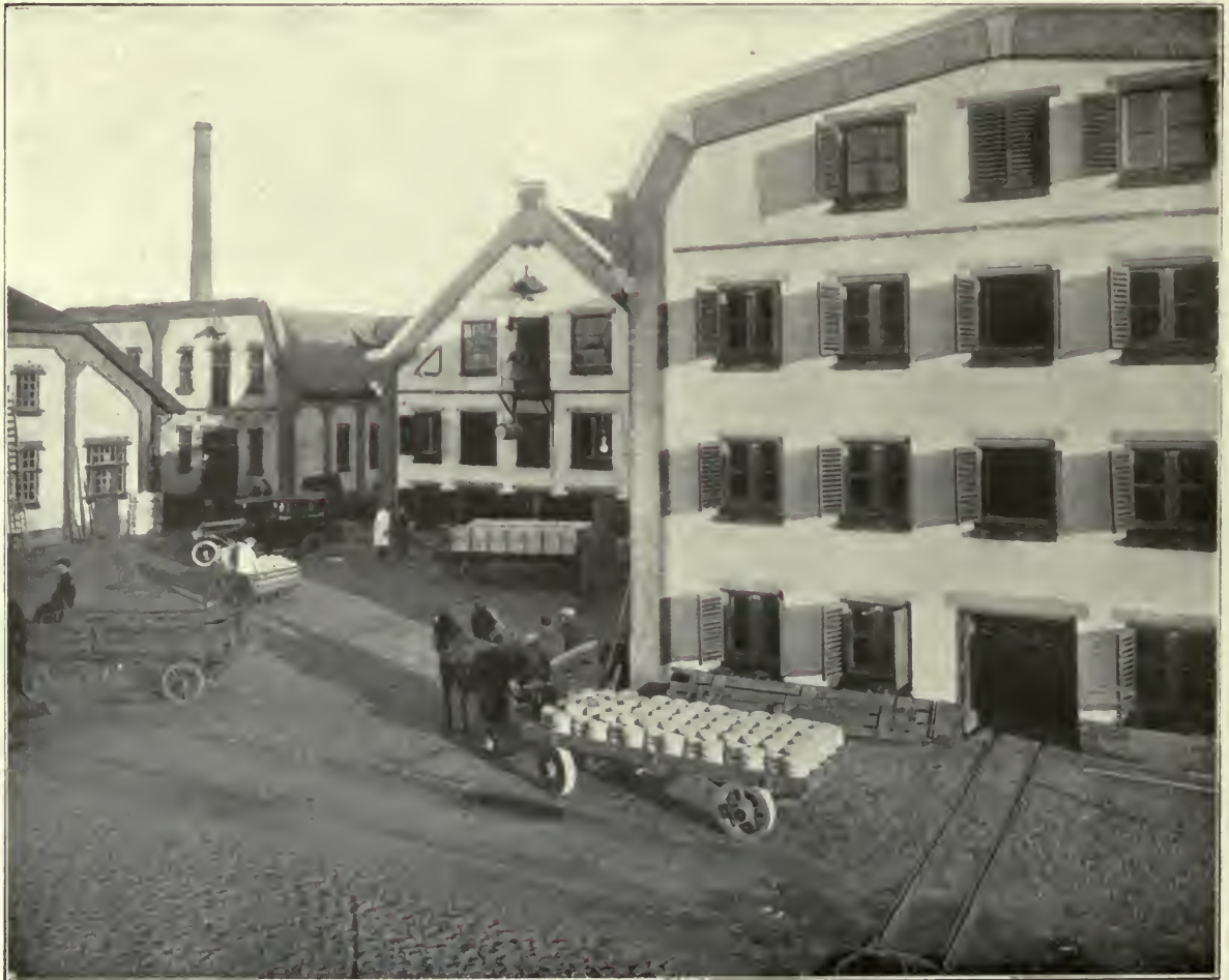
Part of the Central Warehouses at Leeuwarden.
