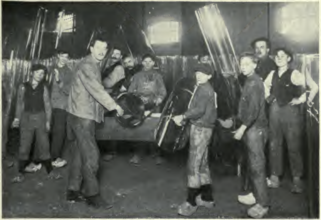
The cooled cylinders are split lengthwise by means of a stick with a diamond inserted in it.
