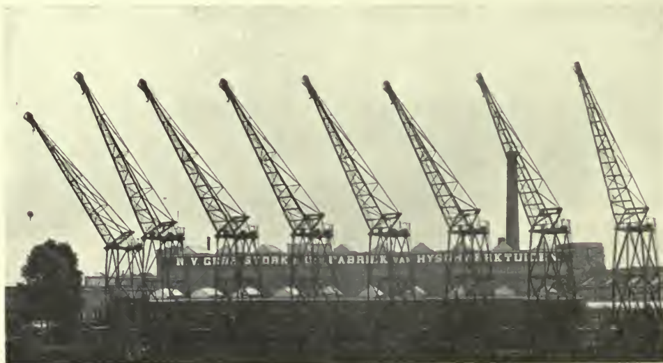
Portal Jib Cranes erected in the Yard of the Hoisting- and Conveying-Machinery Department.
