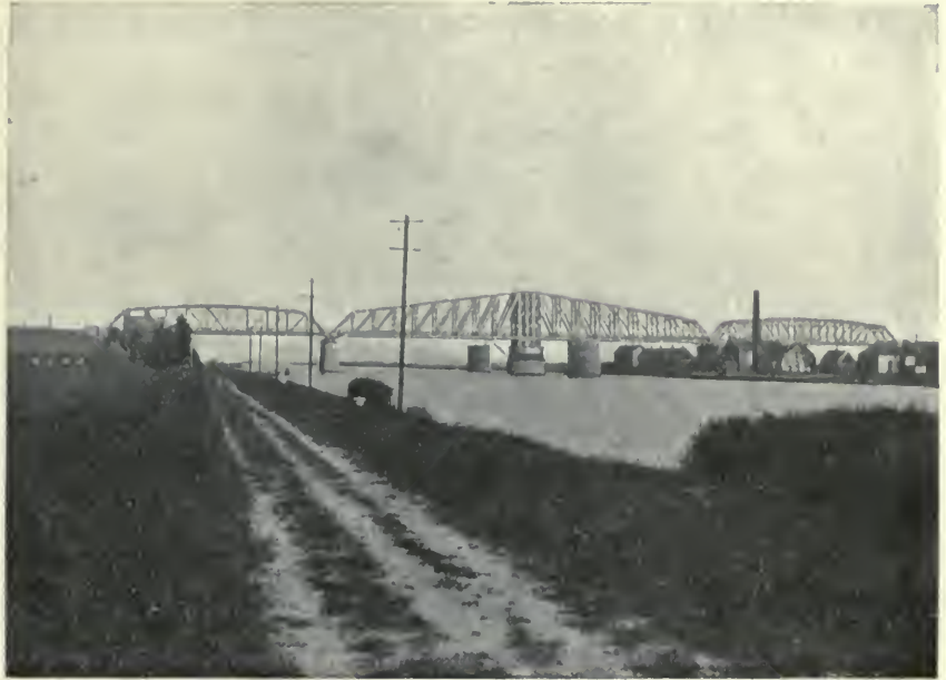
The Hem-Bridge across the North Sea Canal. (The largest swing bridge of Europe).
