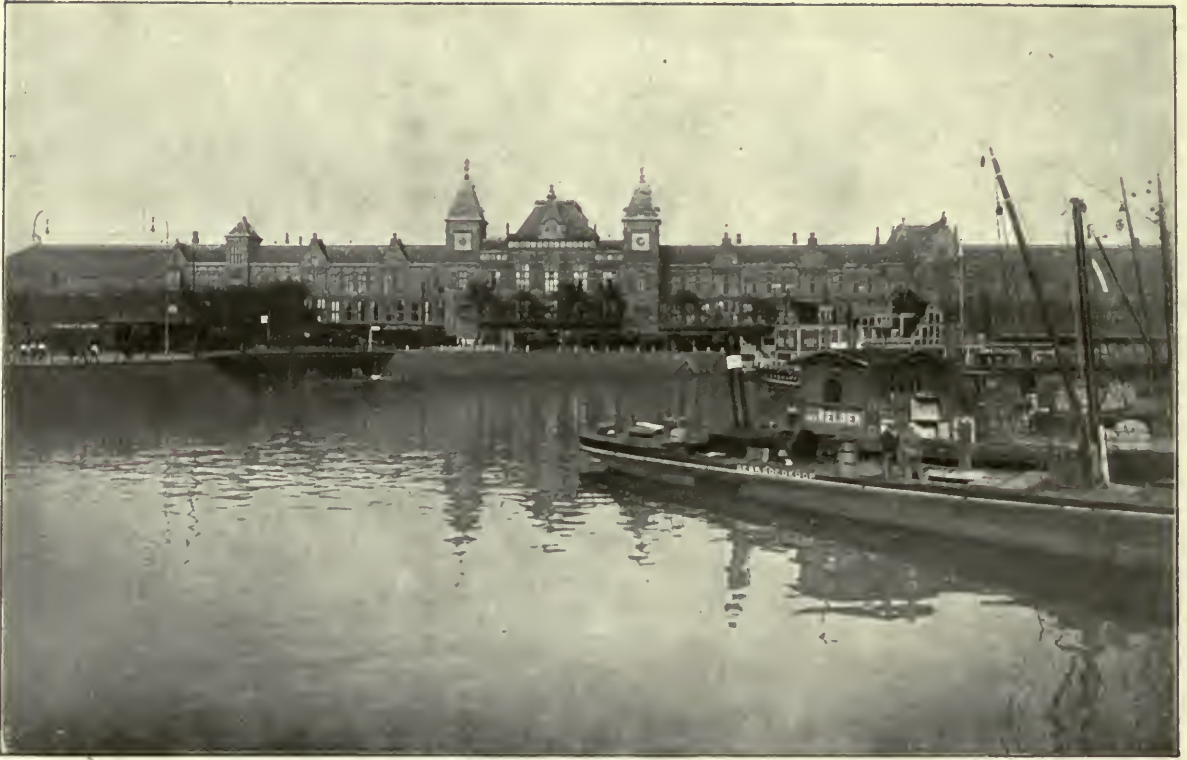
The Central Station at Amsterdam. — Architect Dr. P. J. H. Cuypers.
