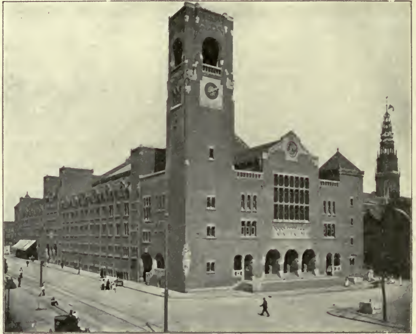
The Exchange at Amsterdam.—Architect Dr. Berlage.
