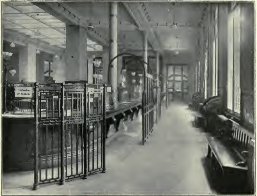
Corner of the Banking Room.
