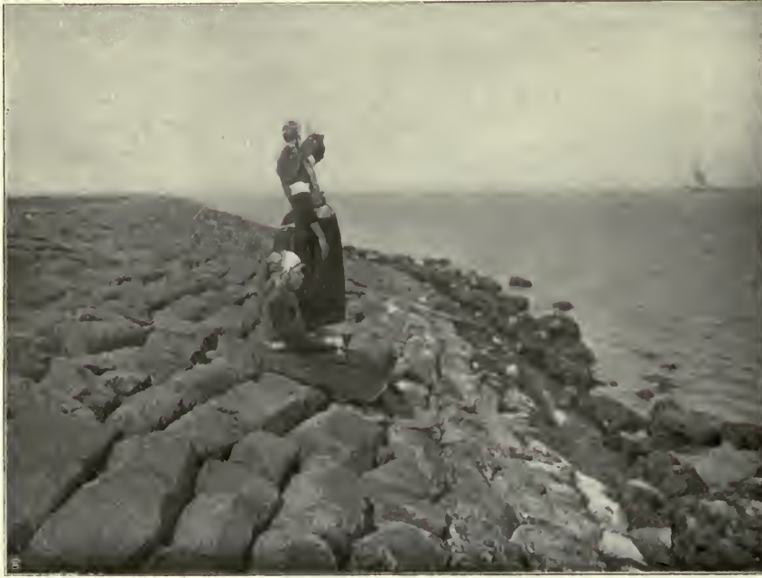
Dike of the Zuider Zee.
