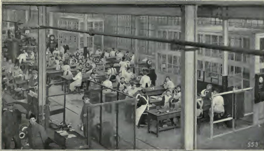
Winding room for small motors.
