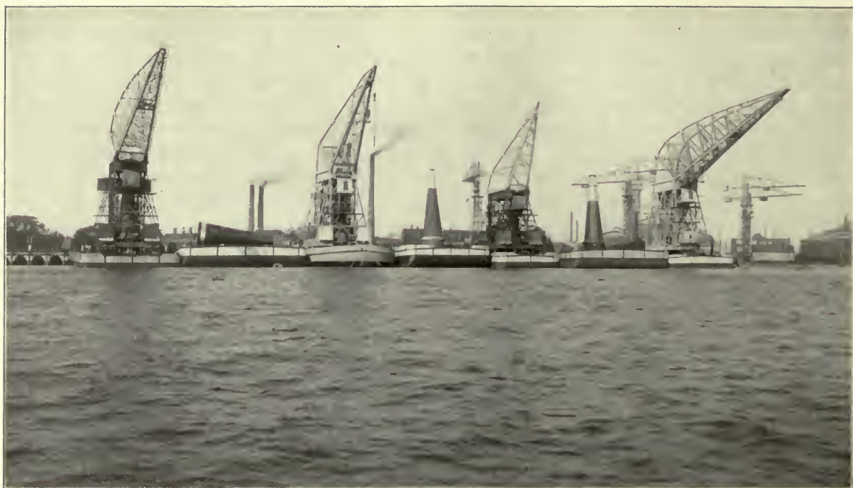
Revolving and derricking cranes in the port of Rotterdam.
