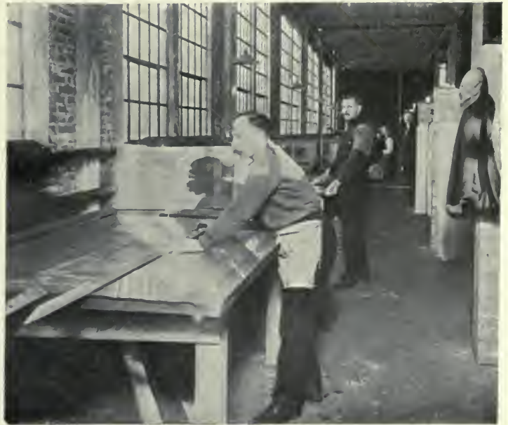
Window panes are cut to measure from the sheets of glass.
