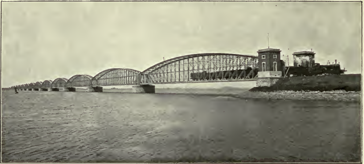
The Bridge across the Moerdijk.
