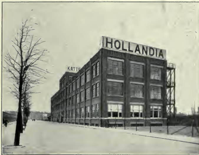
View of the Hollandia Factories.
