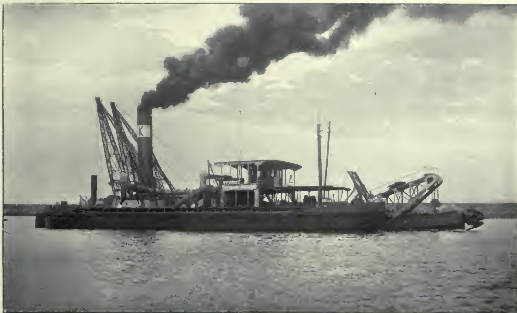
Stationary suction cutter and barge unloading dredger, capacity 6000 tons per hour.
