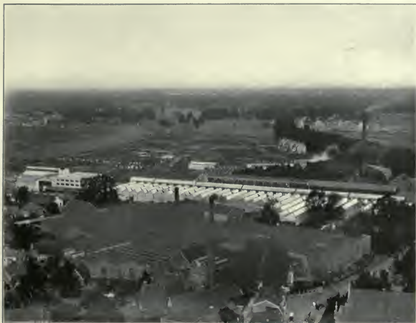
Bird's eye view of the Heemaf Works.
