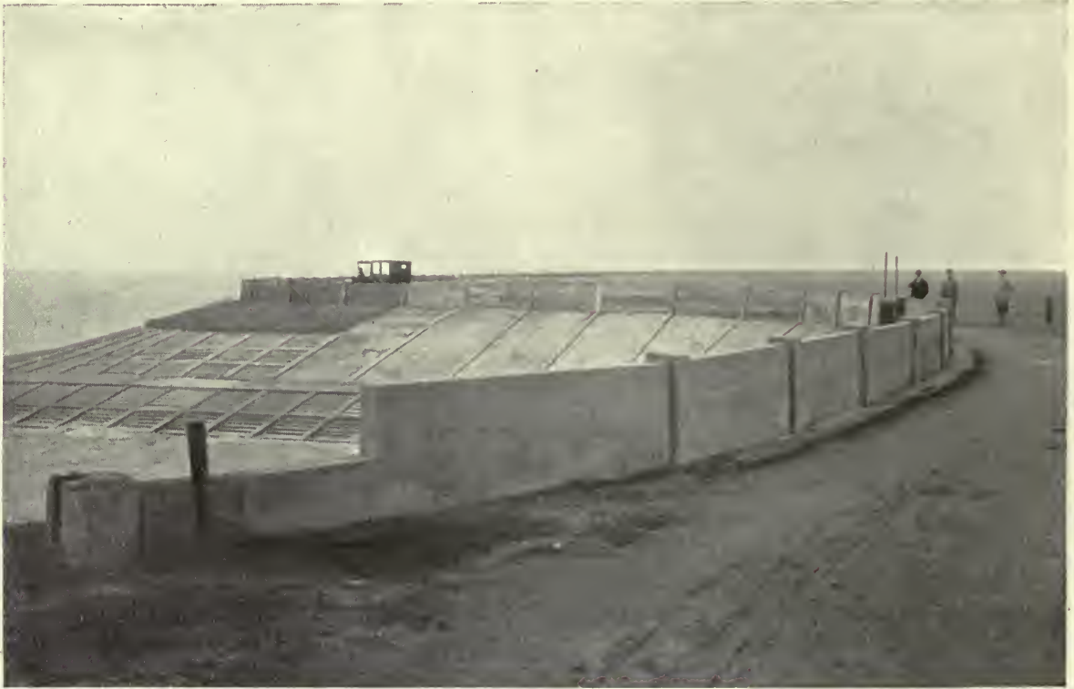
Dike of armoured concrete, de Muralt's system.
