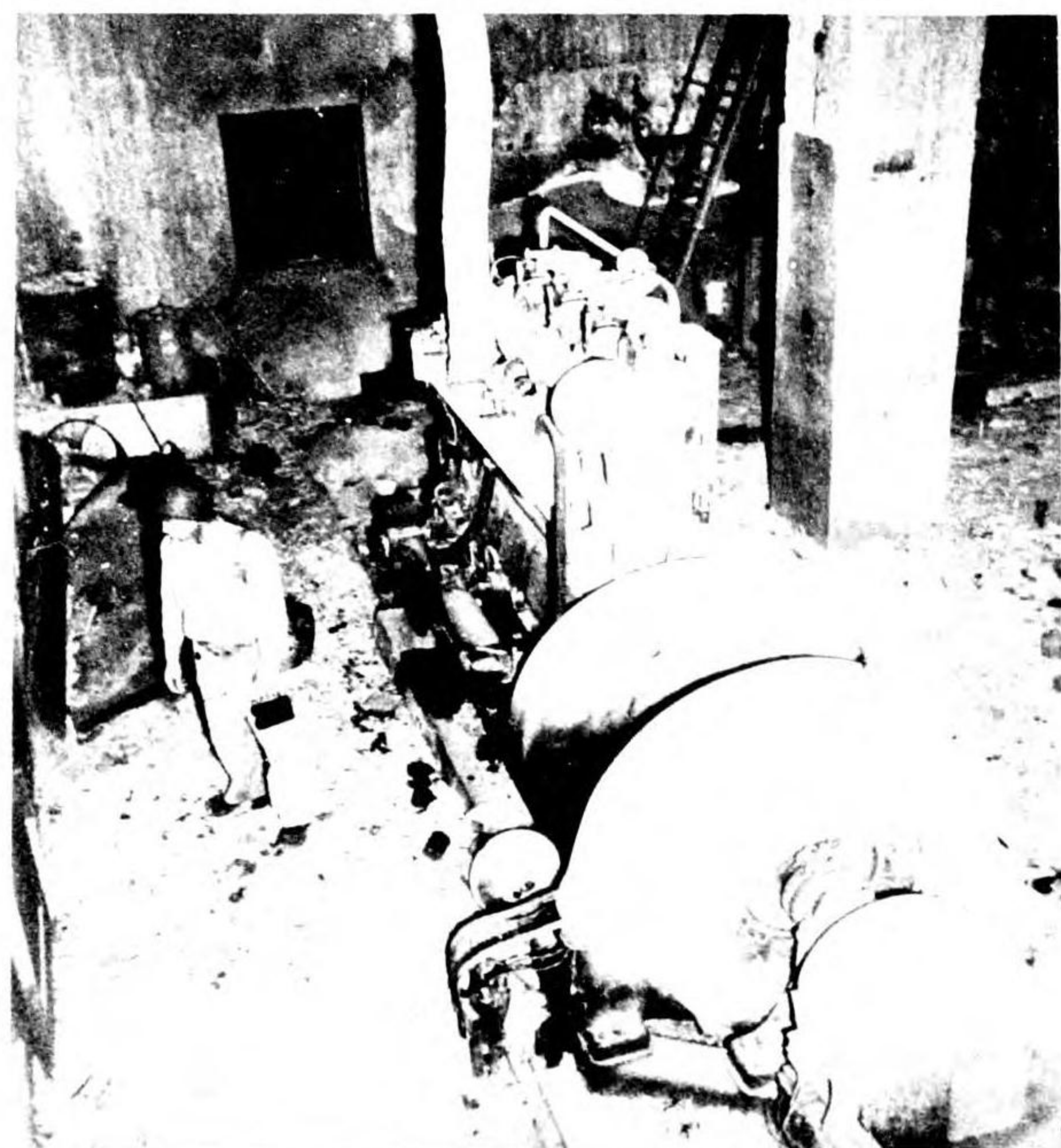
DIESEL GENERATOR - NAMUR
