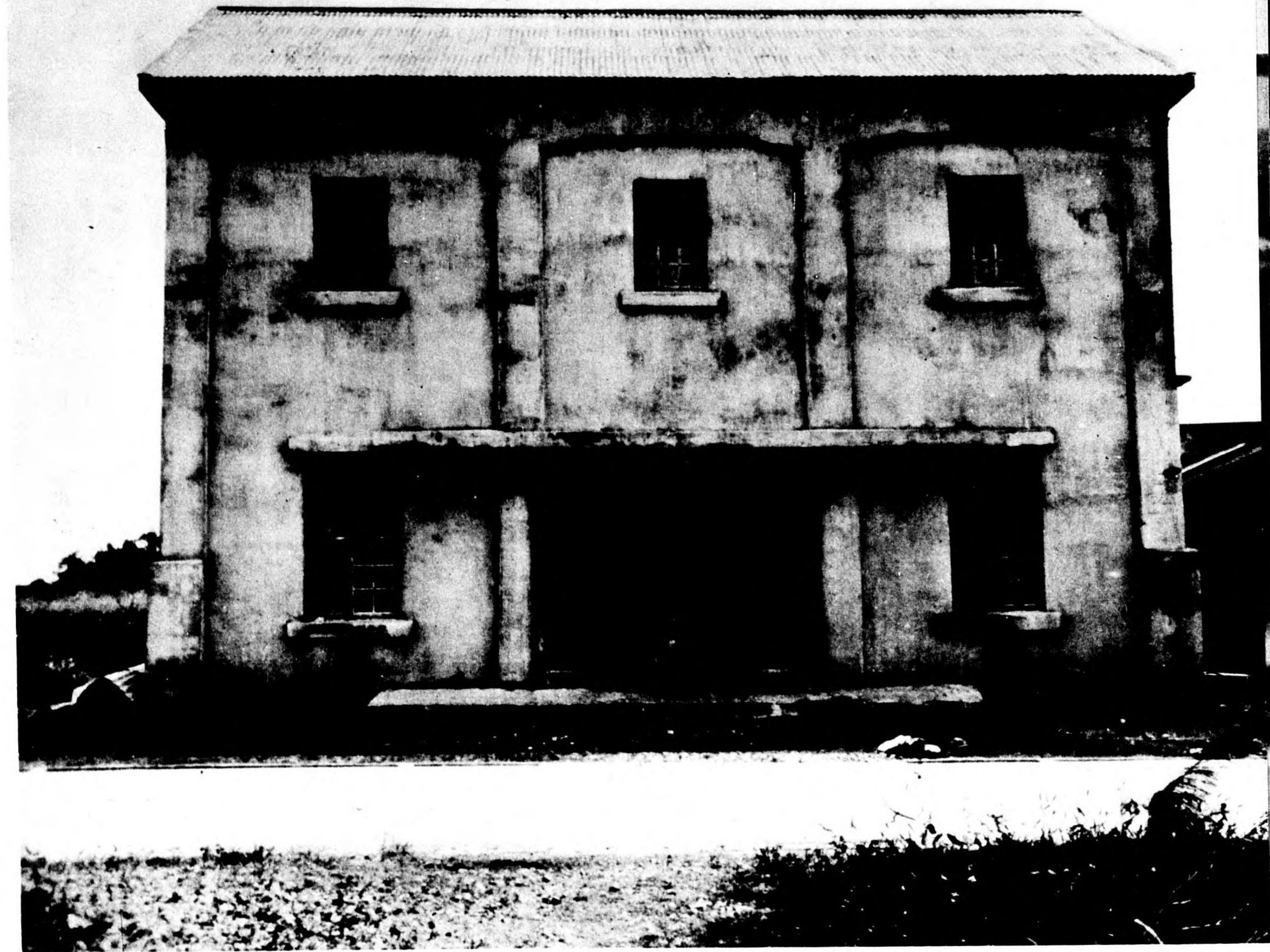
SAIPAN ELEVATION OF CONCRETE POWER DISTRIBUTION STATION
