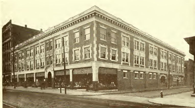
CLINTON HALL AT MAIN AND CLINTON STREETS. One of Springfield's newest hotels, catering to commercial and tourist trade, located three blocks from UNION STATION. Trolley cars for all points can be taken right at the door. There are accommodations for 300 guests. Conducted on the European plan only.
