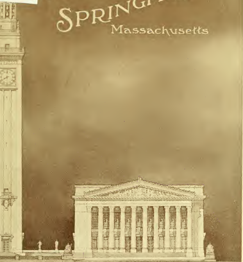
PANICLE MUNICIPAL BUILDING CIVIC CENTER OF SPRINGFIELD
