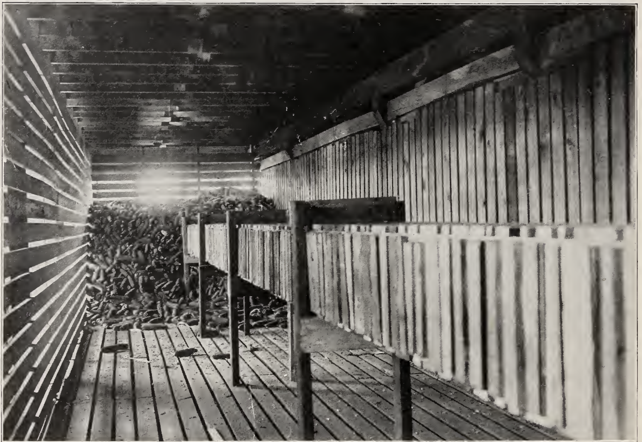
View of Partially Filled Crib, Showing Slatted Air Shaft. Air is Forced to Center of Crib and Out Through Corn.
