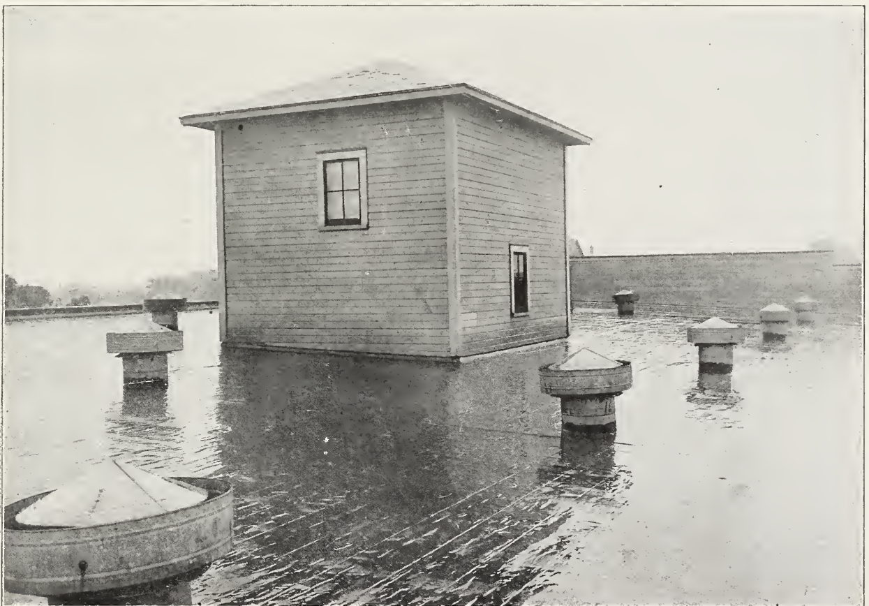
View showing ventilators in roof. These ventilators carry off the moisture on cold, damp days when windows and ventilating doors must be closed.
