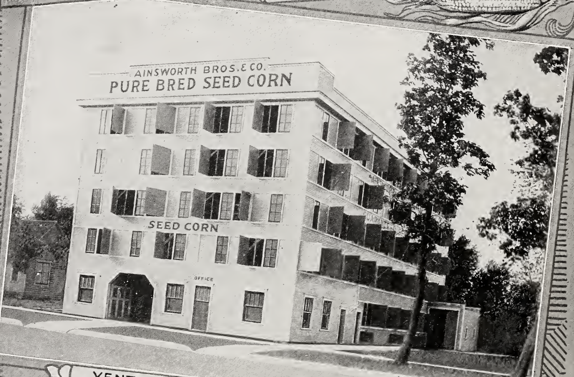
VENTILATING DOORS OPENED
