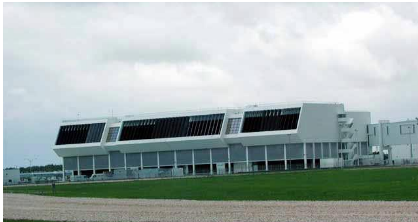
Figure 7-13. Launch Control Center (LCC)
