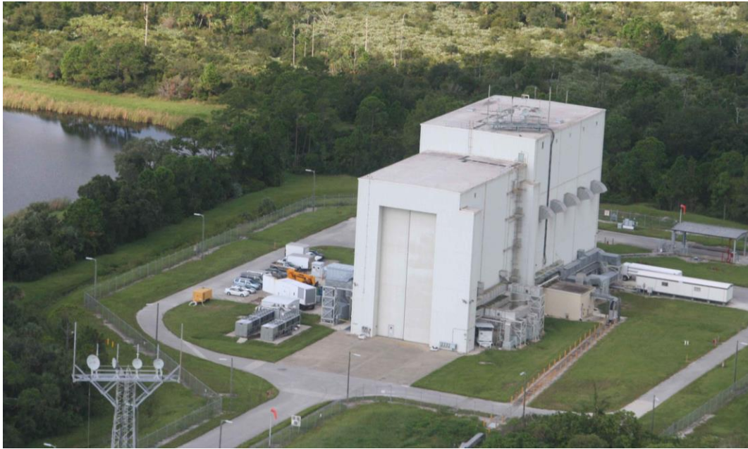
Figure 7-6. Payload Hazardous Servicing Facility (PHSF)
