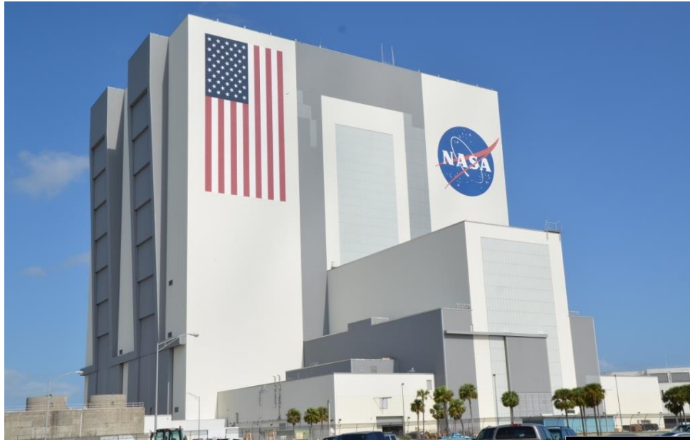
Figure 7-8. Vehicle Assembly Building (VAB)
