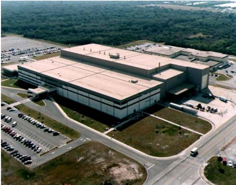
Figure 7-2. Space Station Processing Facility (SSPF)
