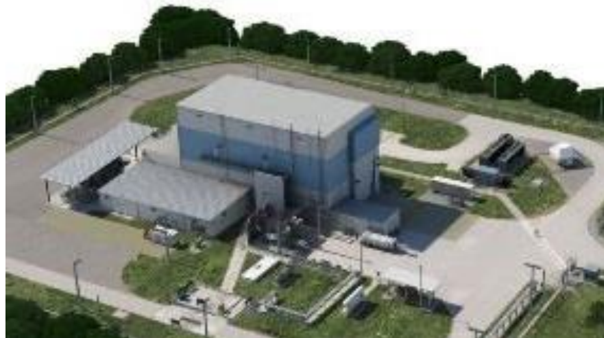
Figure 7-4. Multi Payload Processing Facility (MPPF)
