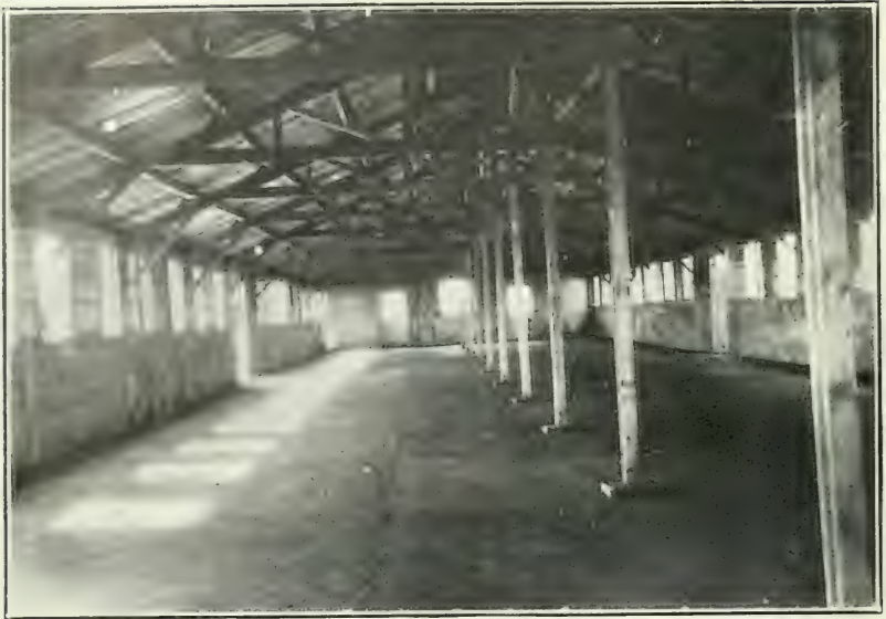
FIG. 3. THE INTERIOR OF THE BUILDING SHOWN IN FIG. 1 BEFORE SUBDIVISION INTO ROOMS.
