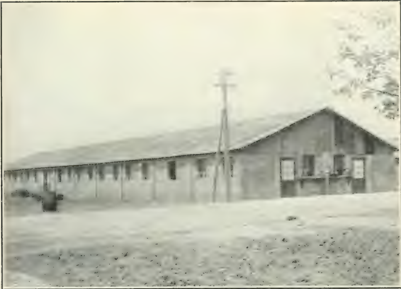
FIG. 1. THE ABOVE PICTURE ILLUSTRATES THE TYPE OF ONE-STORY CONCRETE BUILDING WHICH HOUSED THE VARIOUS DEPARTMENTS OF THE AMERICAN E. F. UNIVERSITY AT BEAUNE, COTE D'OR, FRANCE. IN THE ABOVE BUILDING THE DEPARTMENTS OF BOTANY, PSYCHOLOGY AND ZOOLOGY WERE LOCATED. THESE STRUCTURES WERE APPROXIMATELY FORTY FEET WIDE BY ONE HUNDRED AND SIXTY FEET LONG.
