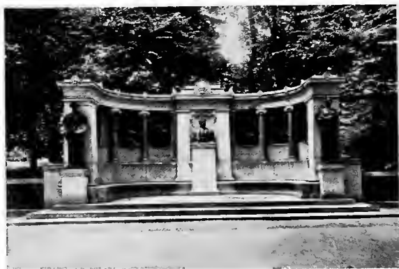
49. Hunt Memorial, by French Post, Architect
