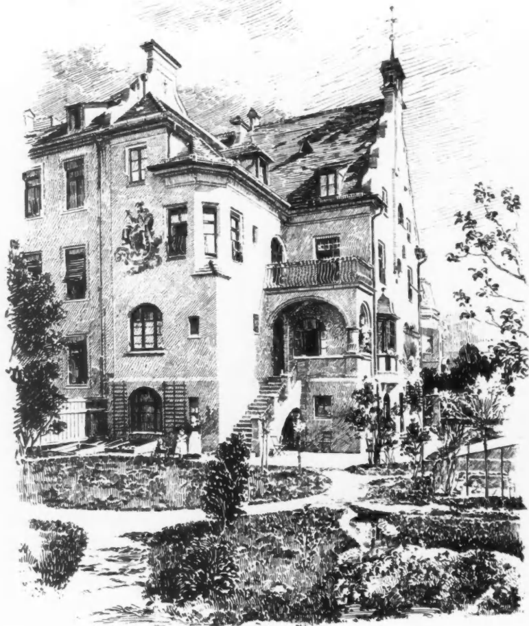
Family House Littmann , M. LITTMANN, Architect, Munich. (For Plans, see p. 122.)
