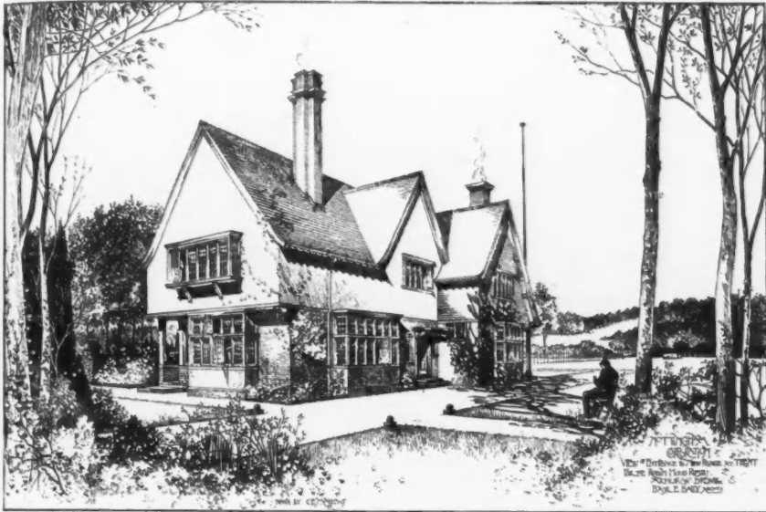
Entrance to New Range at Trent, for the Robin Hood Rifles, BREWILL AND BAILY, Architects.
