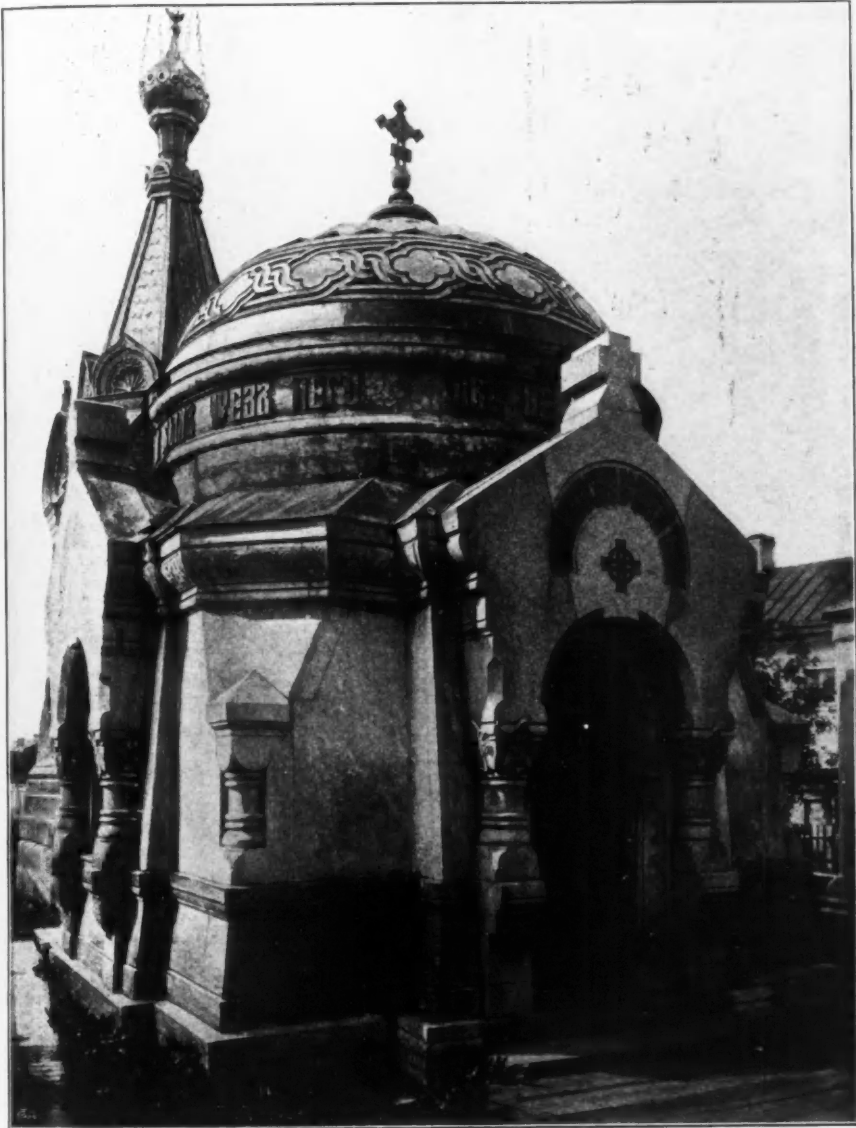
Mausoleum, St. Petersburg, the late M. WALBERG, Architect.
