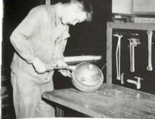
Torque Wrench Application.
