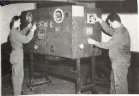
Mockup, Lighting Circuit Wiring.
