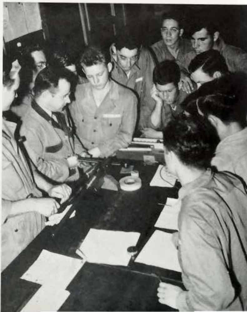
Swaging Terminus on Control Table.
