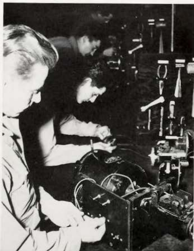
Coil Test Stand.
