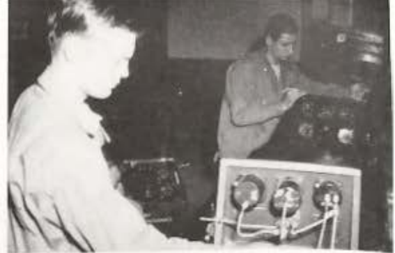
Mockup, Pilot Static System.
