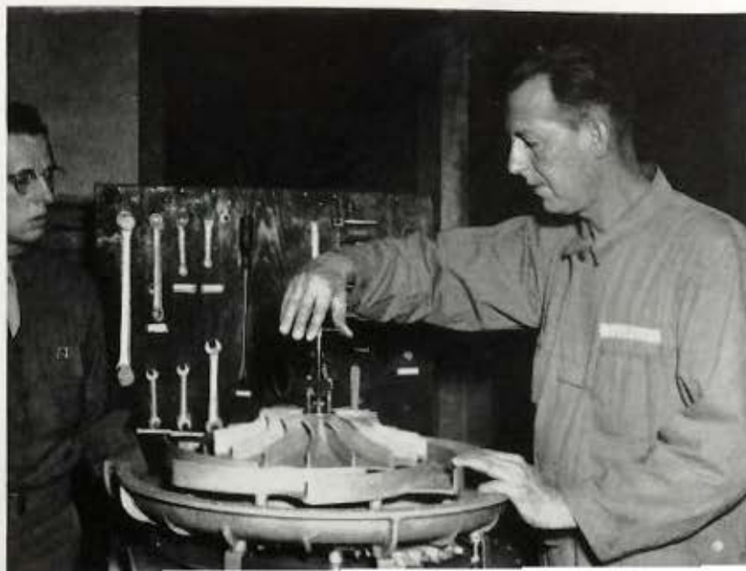
Impeller Puller Tool.
