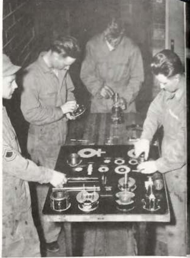
Starter-Energizer Parts Rack.
