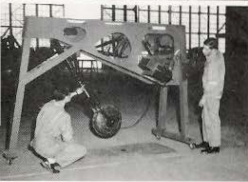
Mockup, Warning and Limit Switches System.
