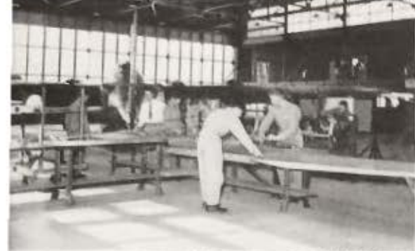
Repairing Wing Flaps.
