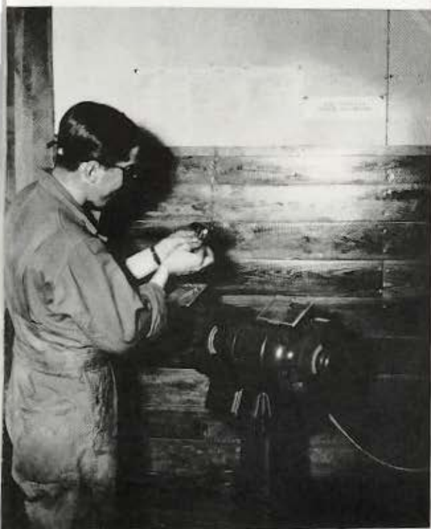
Drill Pitch Checking.
