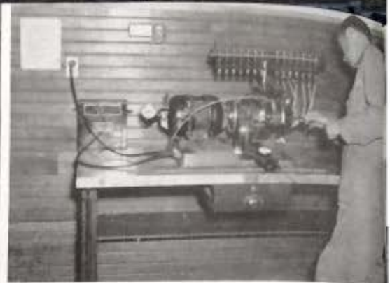
Magneto Test Stand.
