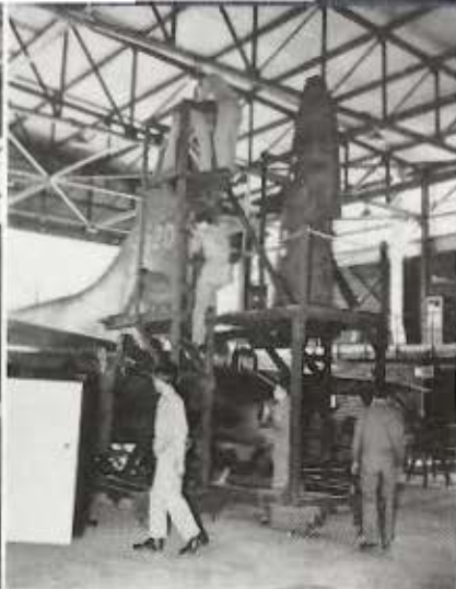
Removing Tail Assembly.
