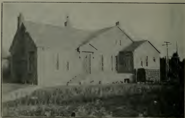
An attractive peninsula home of substantial construction— Burlingame, San Mateo County.
