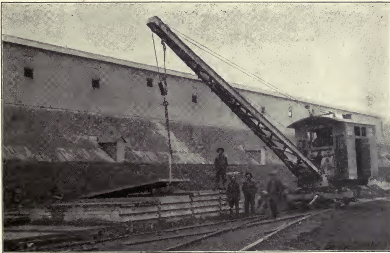
Fig. 245.—View Showing Method of Handling Roof Slabs.
