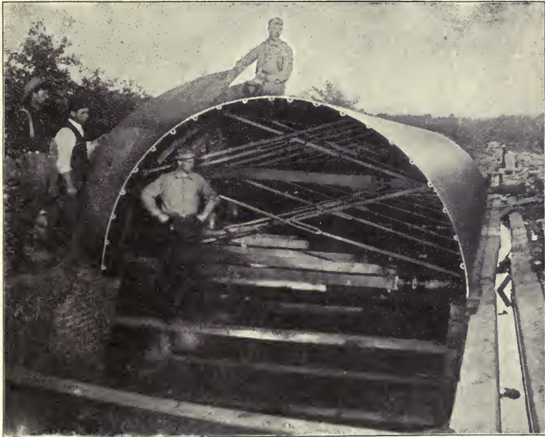
Fig. 247.—Blaw Collapsible Steel Centering for Conduit Construction.
