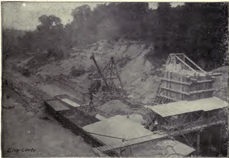
Fig. 140.—View of Mixer Plant Showing Method of Unloading Materials, Burton Tunnel.
