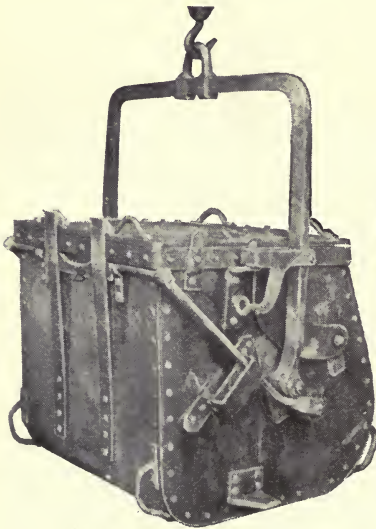
Fig. 27.—Cyclopean Bucket for Depositing Concrete Under Water (Closed Position).
