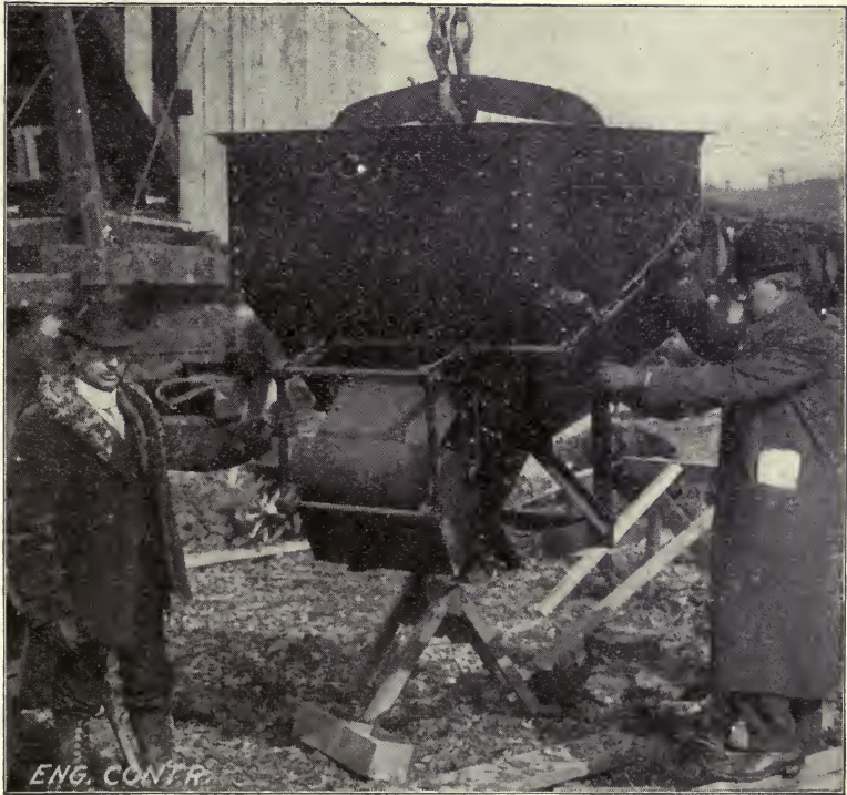
Fig. 222.—Special Concrete Bucket for Large Warehouse Building.
