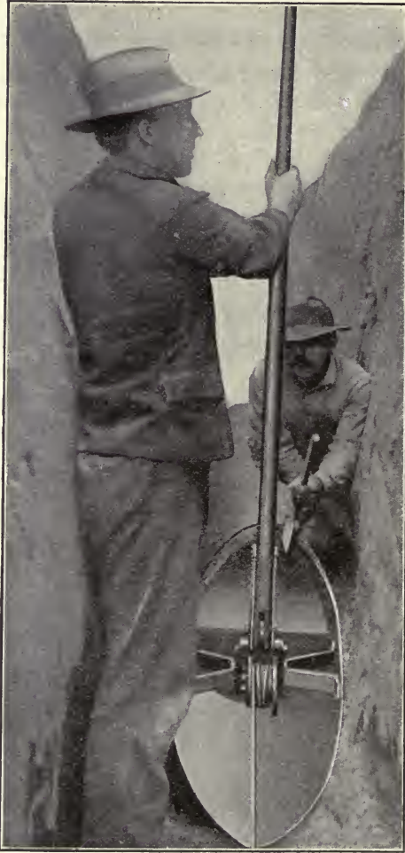
Fig. 268.—Ransome Continuous Mold for Concrete Pipe Construction.
