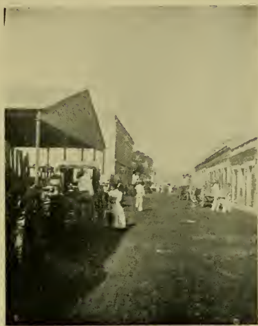
Street at the Bay, Ponce.
