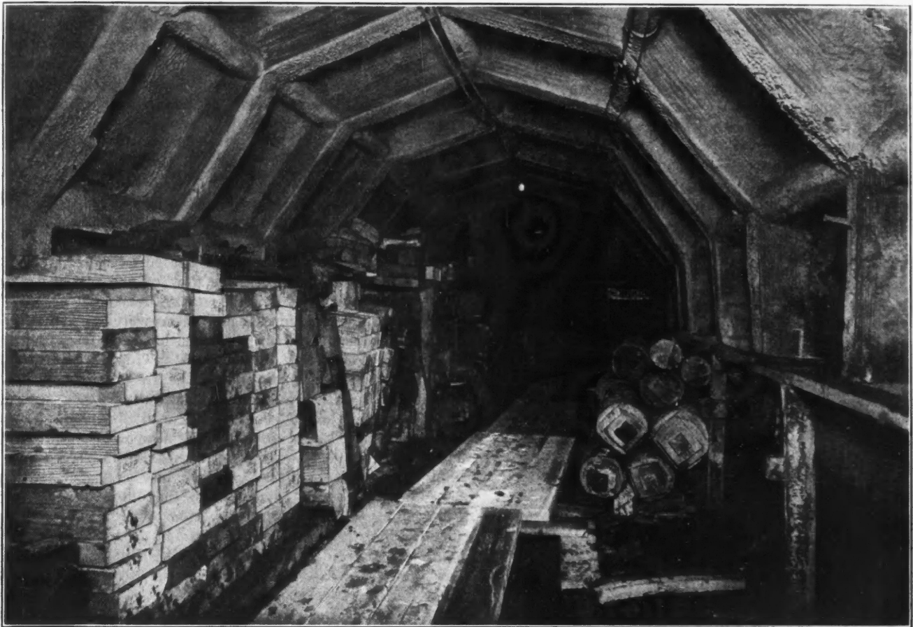
TIMBER STATION AT 2,800-FT. LEVEL OF SPECULATOR MINE, BUTTE, MONT.
