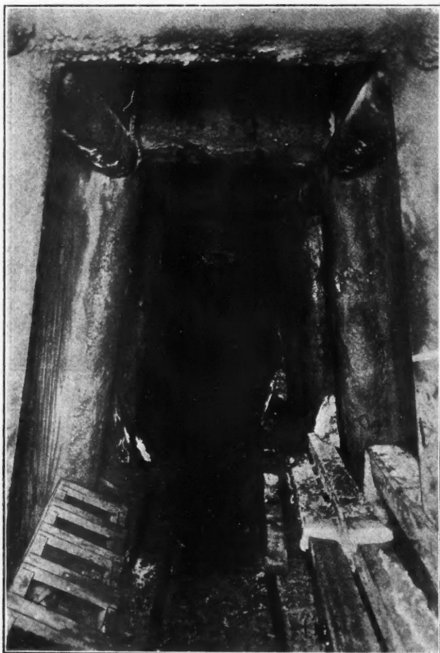
CEMENT-TREATED TIMBER IN A CROSSCUT
