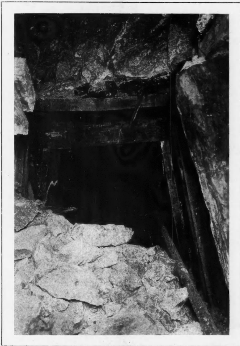
A TYPICAL CAVE-IN Drift in Copper Mine in Butte District, Montana
