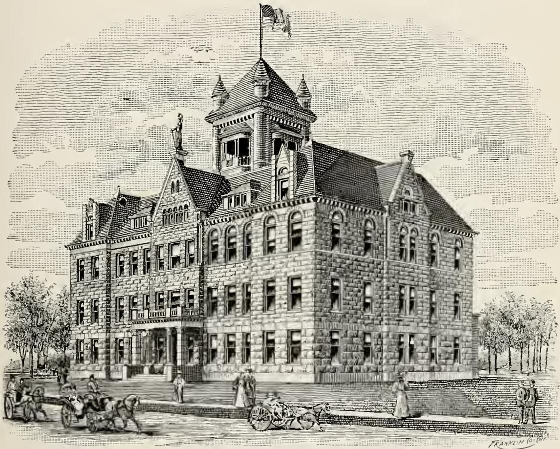
MONROE COUNTY COURT HOUSE
