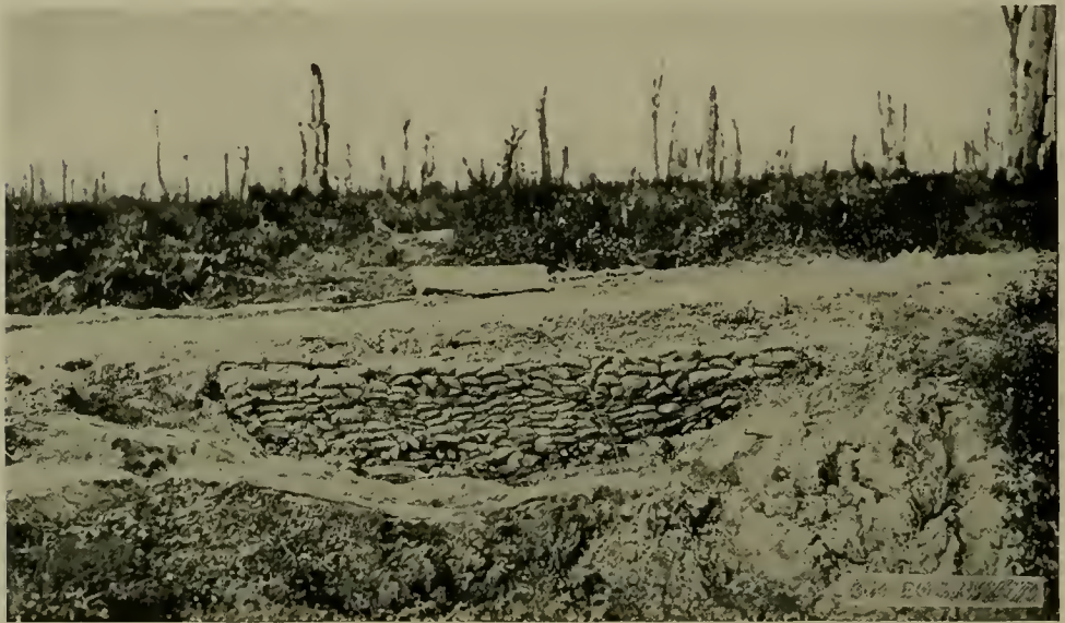
ROAD OVER NO-MAN'S LAND, RECONSTRUCTED BY 304 ENGRS., SHOWING METHOD OF FILLING SHELL HOLES.
