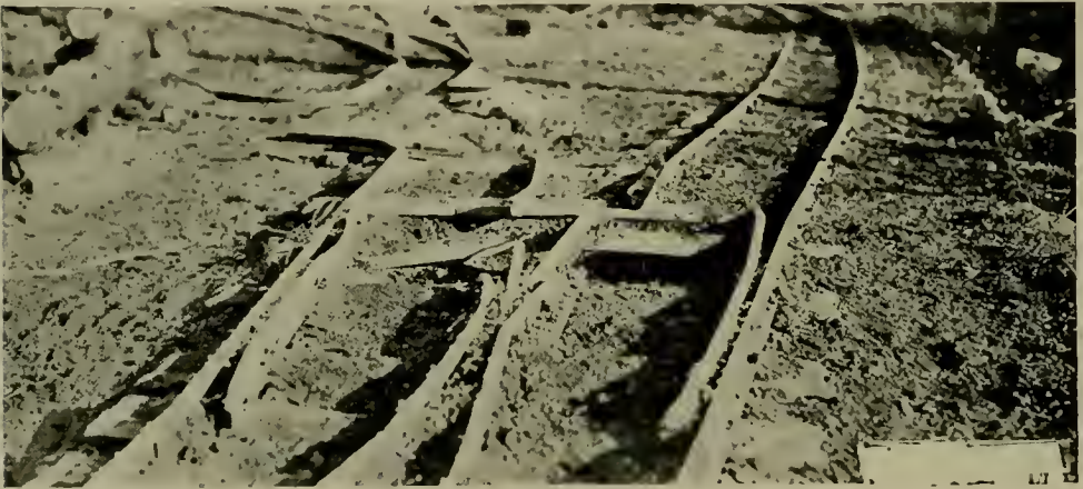
BROKEN RAILROAD TRACKS NEAR MOLLEVILLE FARM.
