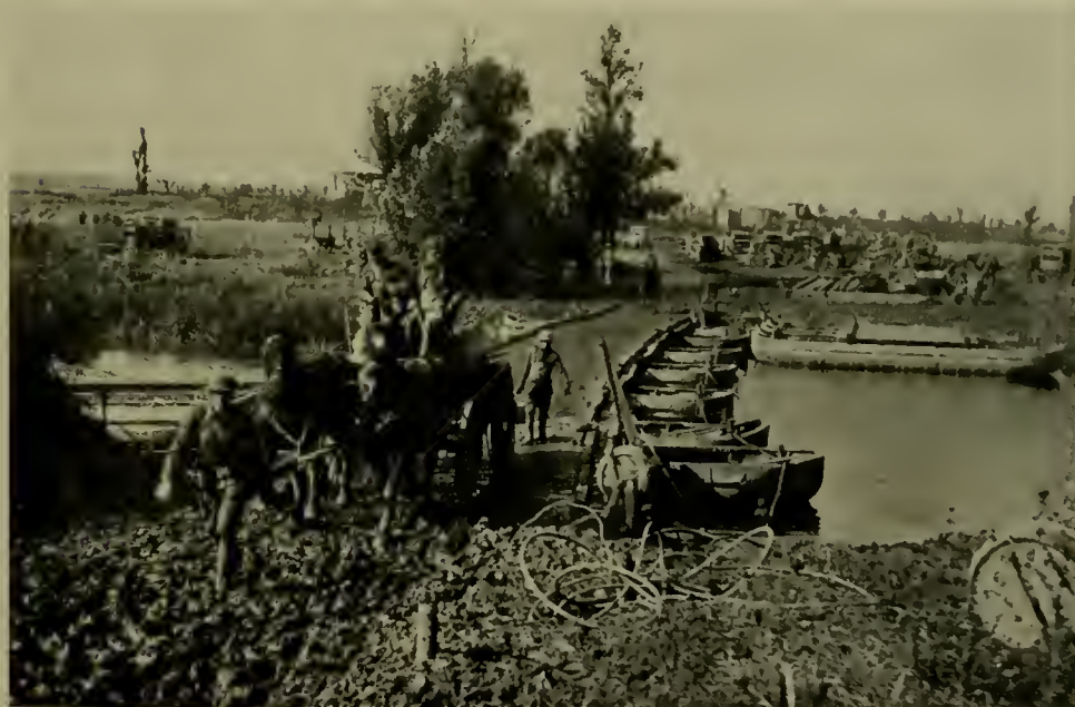
FRENCH PONTOON BRIDGE ACROSS THE MEUSE CONNECTING REGNEVILLE AND SAMOGNEUX.
