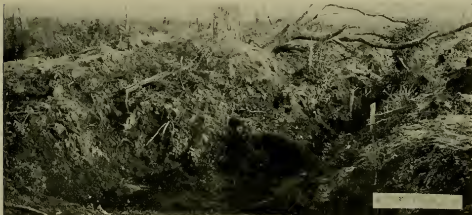
DEMOLISHED GERMAN TRENCH, IN THE BOIS DE MONTFAUCON.
