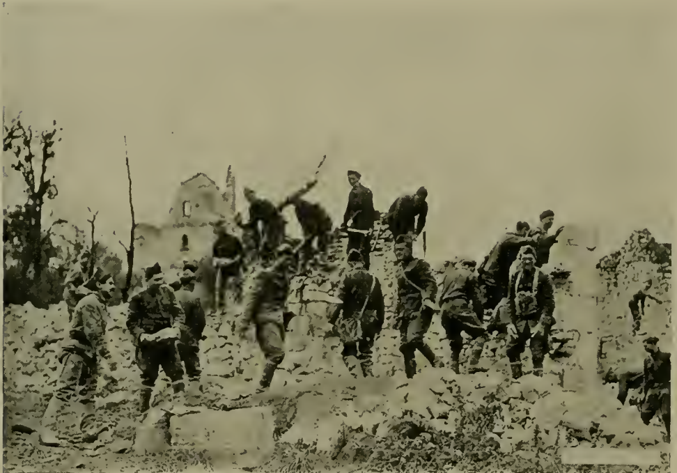
DEMOLISHING WALLS FOR ROAD-BUILDING STONE—ST. REMY-TROYON SECTOR.
