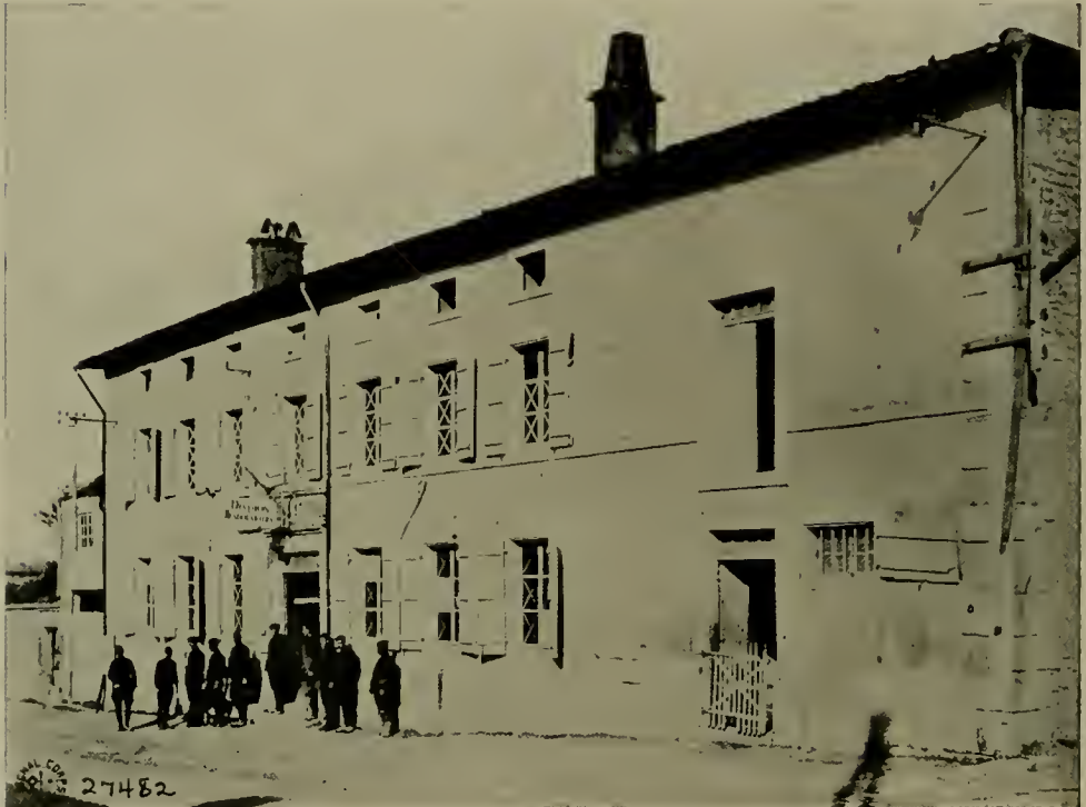
HOTEL DE VILLE, TROYON-SUR-MEUSE, 79TH DIVISION HEADQUARTERS OCT. 8-28, 1918.
