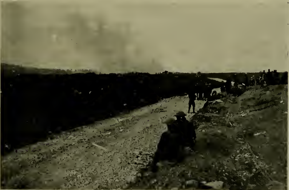
BOX BARRAGE, EVENING OF OCT. 30, 1918, ON THE EDGE OF BOIS DE CONSENSVOYE. NOTE DELAYED TRAFFIC AND OUR GUNS UNDER CAMOUFLAGE ON THE RIDGE
