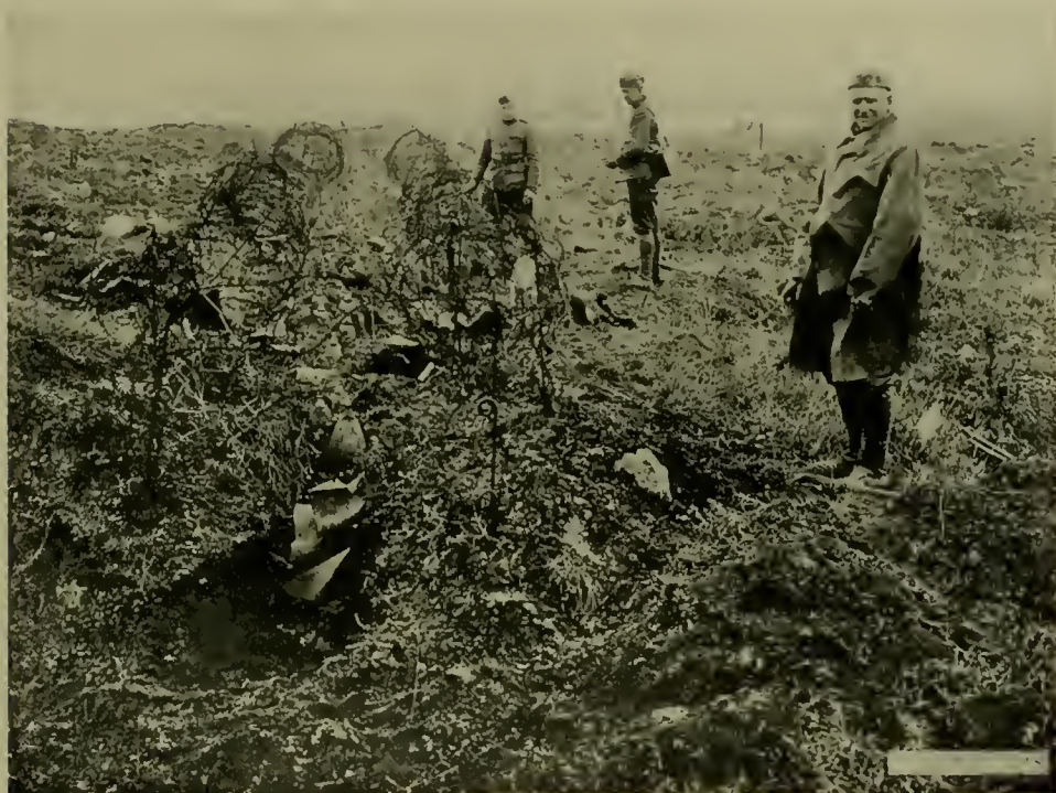
304TH ENGINEERS REMOVING TANK BARRIER EAST OF DAMVILLIERS.
