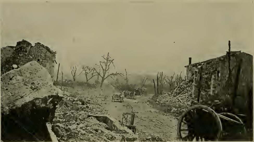
STREET IN MONTFAUCON LOOKING TOWARD FAYEL FARM.
