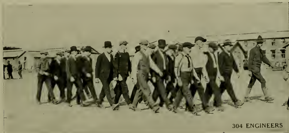
NEW MATERIAL GOING TO BE OUTFITTED
