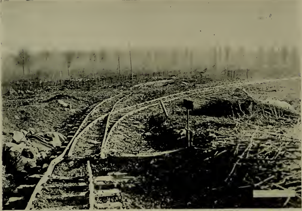
EFFECT OF SHELL FIRE ON NARROW GAUGE RAILROAD ON CREST OF HILL ABOVE MOLLEVILLE FARM, DEAD BOCHE BESIDE THE TRACK.
