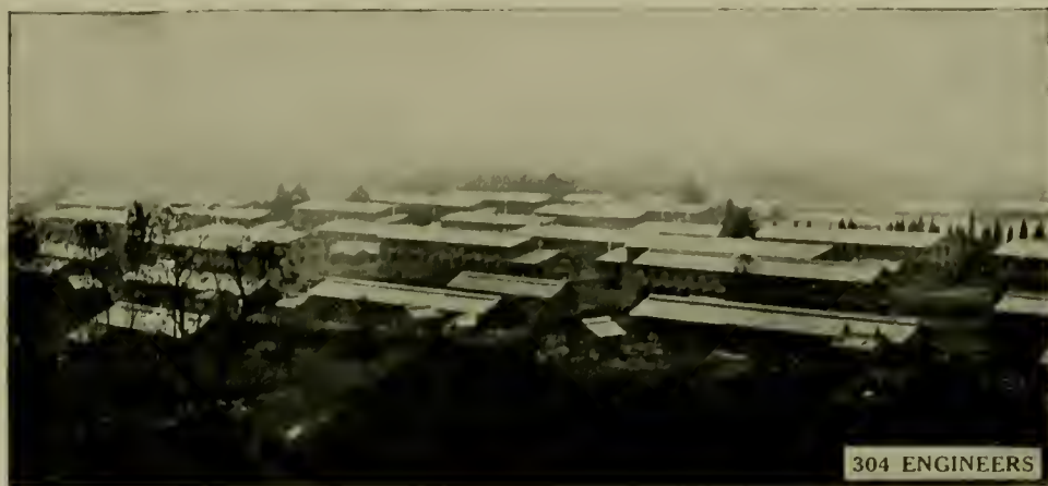
BIRD'S-EYE VIEW OF THE CANTONMENT FROM DIVISION HEADQUARTERS
