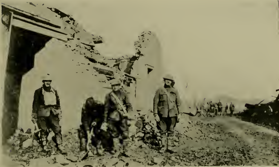
MEN OF THE 304TH ENGINEERS REPAIRING ROAD IN DAMVILLIERS. MACHINE GUN BULLETS WERE CRACKING OVER THEM WHEN THIS VIEW WAS SNAPPED
