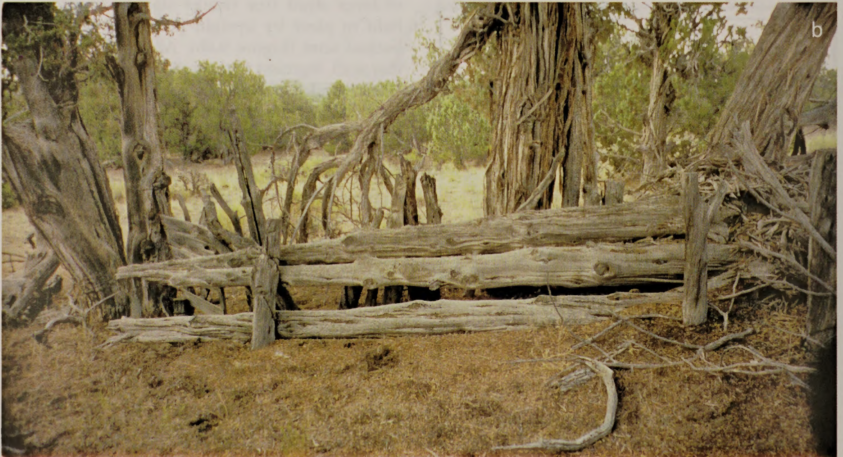
Figure 9.6. Corral at 42KA4546 on Long Flat; a) detail of wall construction; b) wall construction at junction of three lobes.
