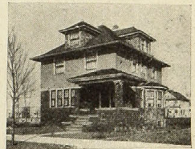
A No. 4121 IDEAL Boiler and 420 ft. of 38-in. AMERICAN Radiators, costing the owner $190, were used to Hot-Water heat this cottage.
