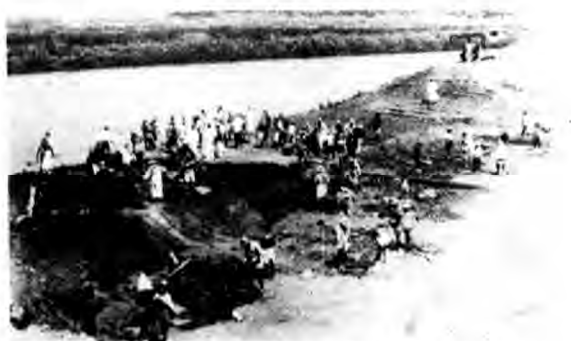
形情工施程工築翻松里八汎郵高程工復復河運
