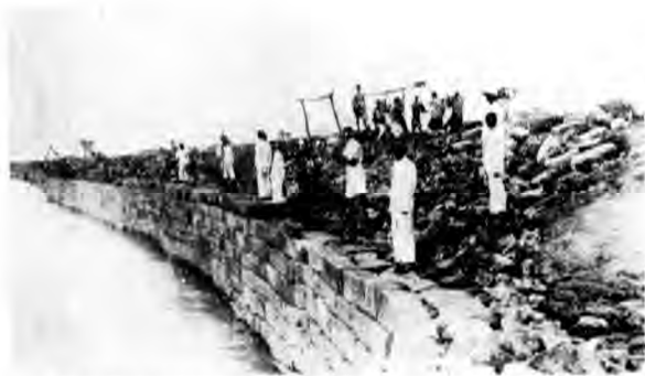
形情工施程工石餘荷海北南塘家萬汎郵高程工復復河運
