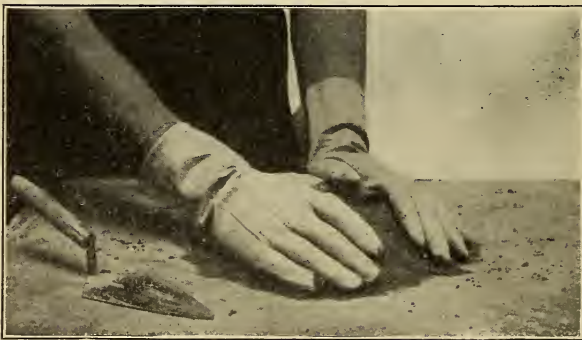
FIG. 51.—Making Briquettes—Kneading.
