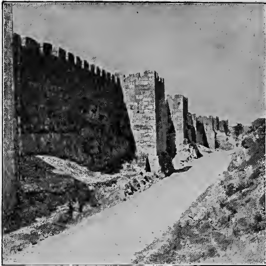
WALL WITH ABUTMENTS AT JERUSALEM.
