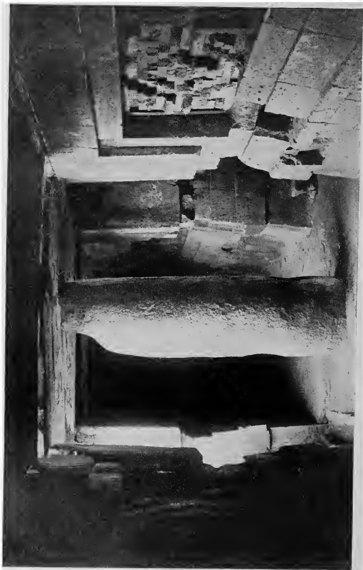
BASEMENT GALLERIES AND COLUMNAR ROOF SUPPORT AT MITLA. Courtesy of the Field Columbian Museum.
