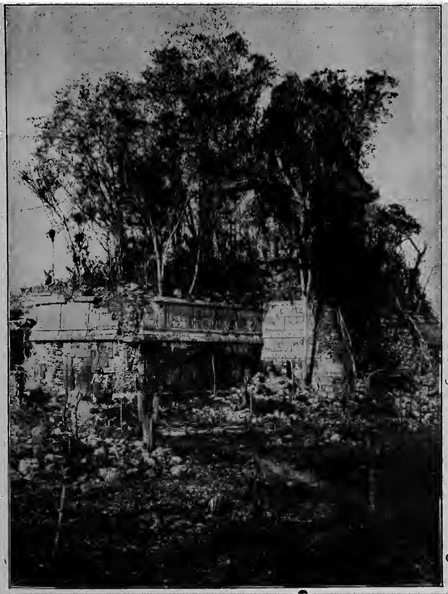
RUINED PALACE AT XKICHMOOK—THE NORTHWEST.
