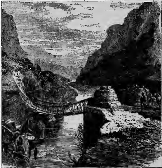
SUSPENSION BRIDGE OVER RIO PAMPAS.
