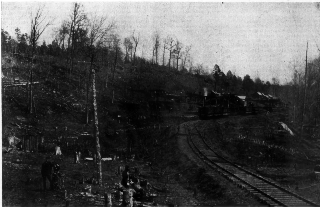
PLATE 1.—VIEW OF THE TANNEHILL BROWN ORE DEPOSIT (GOETHITE), TUSCALOOSA COUNTY, ALABAMA, AT THE BEGINNING OF MINING IN 1887.
