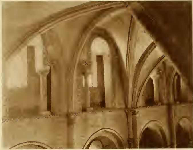
FIG. 61. S.-Etienne, Caen, (Calvados). Nave vaults.
