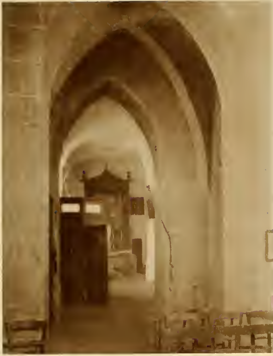
FIG. 13. Crony-sur-Oureq. (Seine-et-Oise). Vault under Tower.
