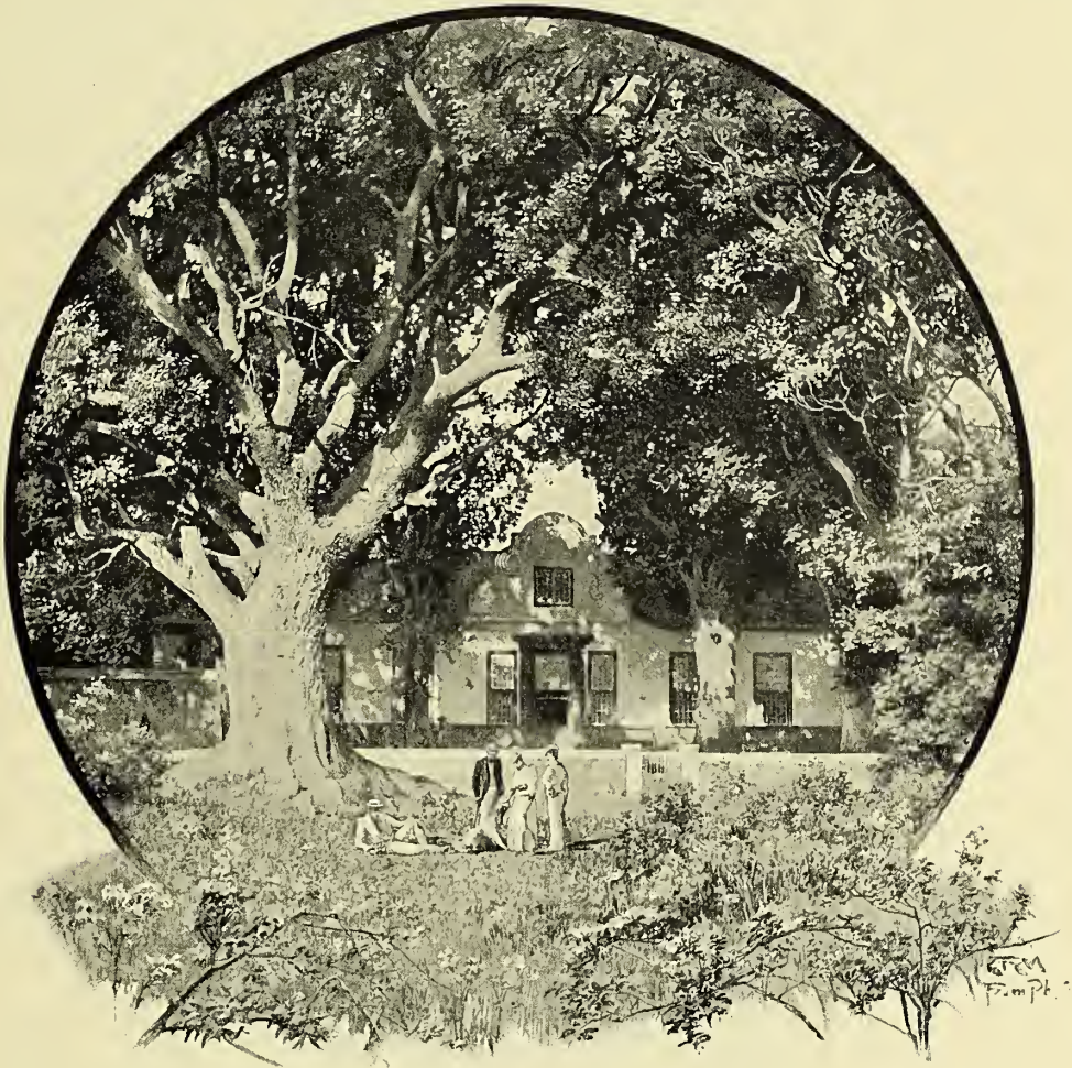
CAPE TOWN RESIDENCE OF THE PRESENT DAY.
