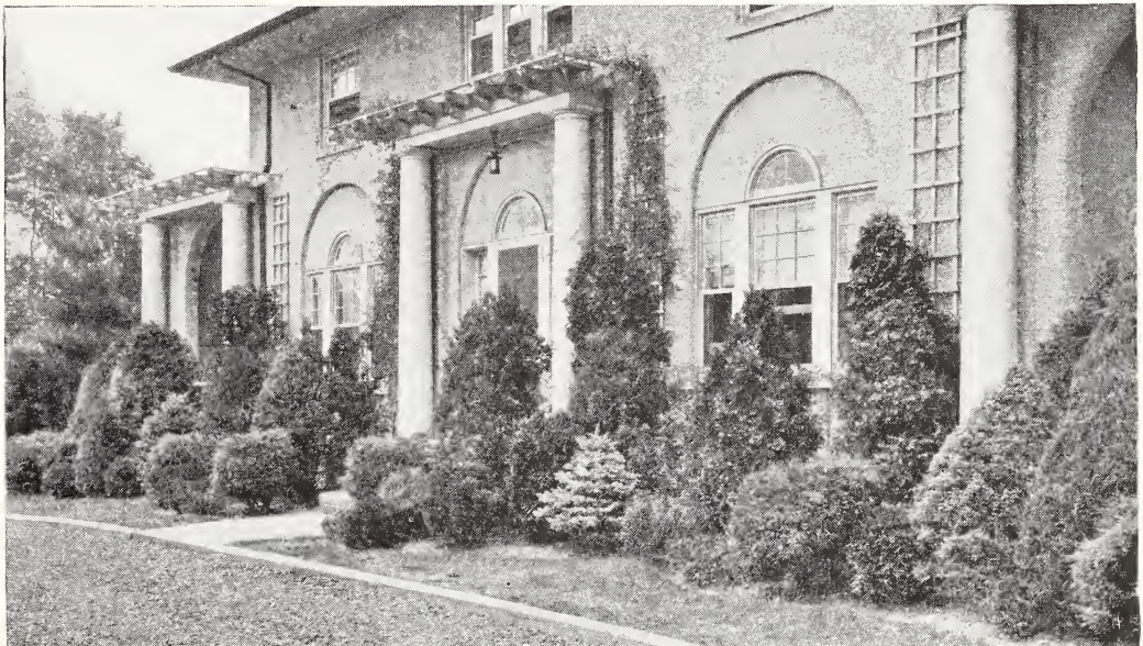
Evergreens give a restful appearance to the home
