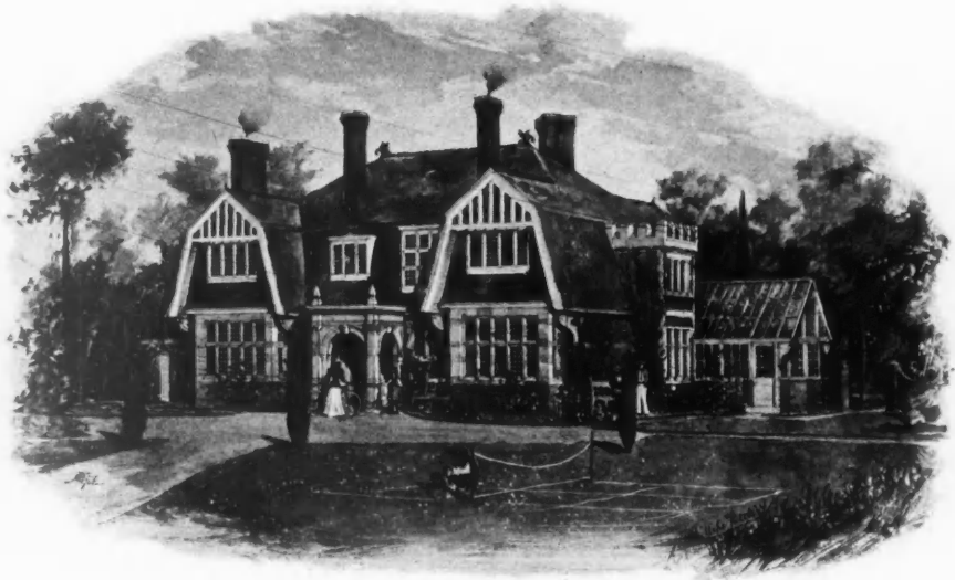
A Country House in Surrey , H. PHILLIPS FLETCHER, A.R.I.B.A., Architect. (For Plans, see p. 87.)
