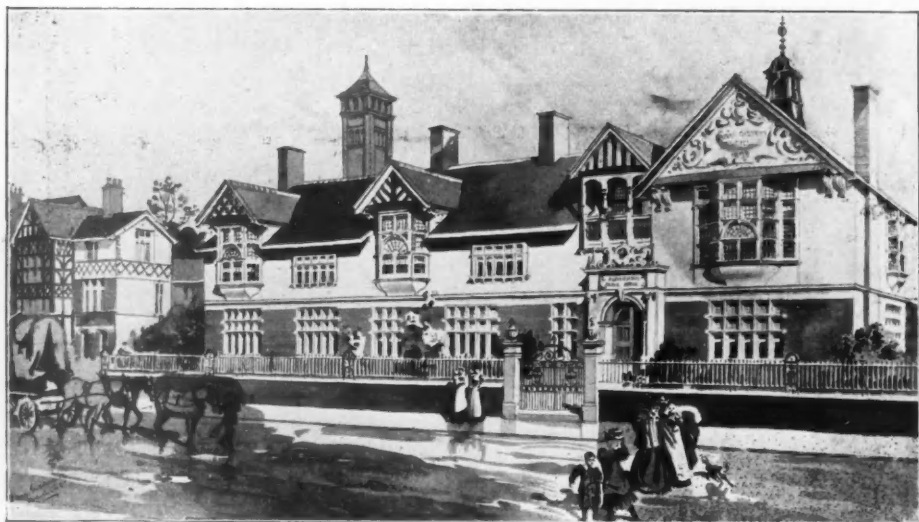
1729. Altrincham Council Offices , HENRY GOLDSMITH, Architect. (For Plan, see p. 104.)
