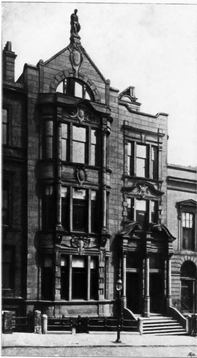
703. Business Premises, St. Vincent Street, Glasgow, FRANK BURNET AND BOSTON, Architects.
