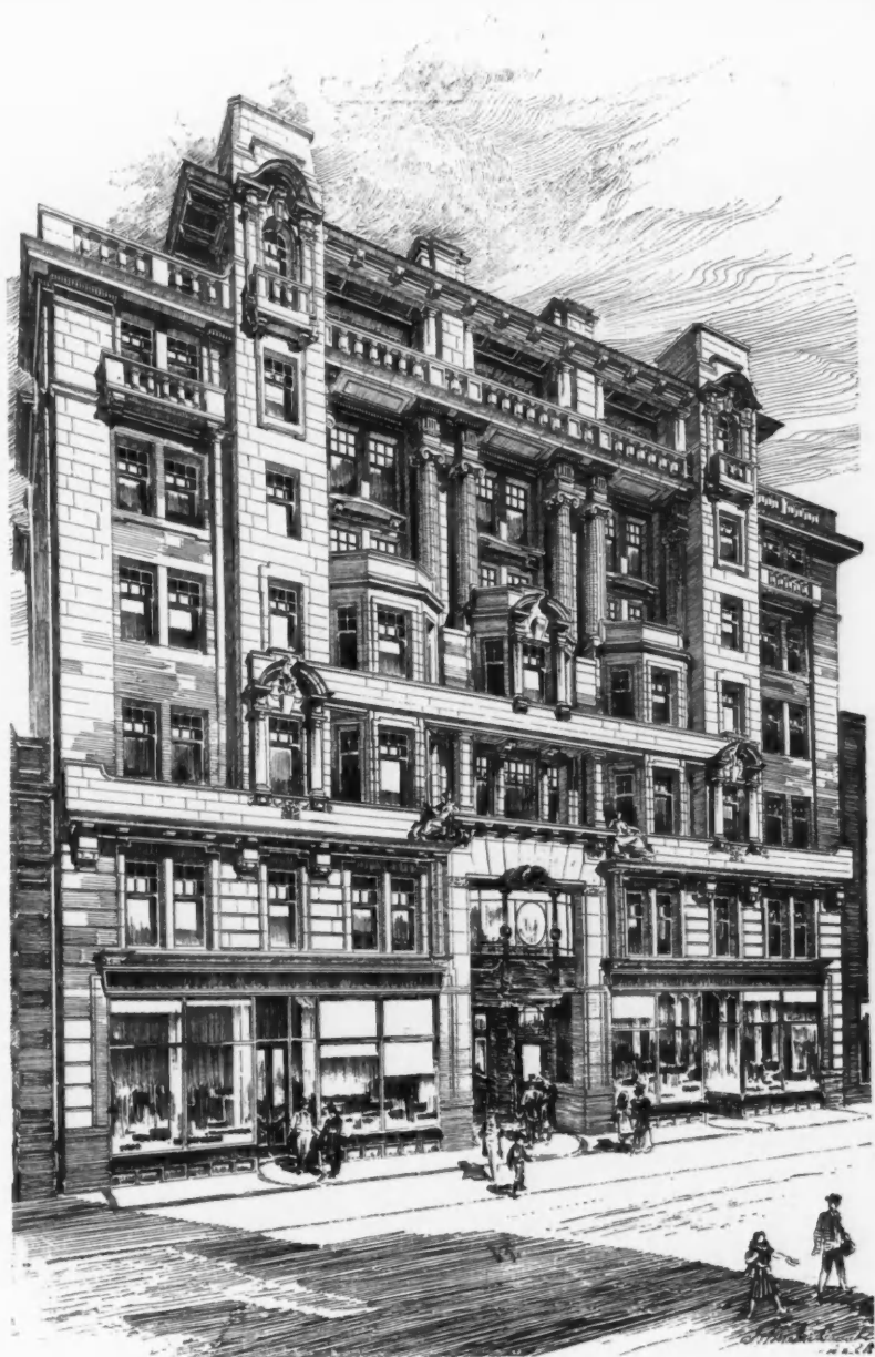
749. Waterloo Chambers, Glasgow , JOHN JAMES BURNET, A.R.S.A., Architect. (For Plans, see p. 104.)
