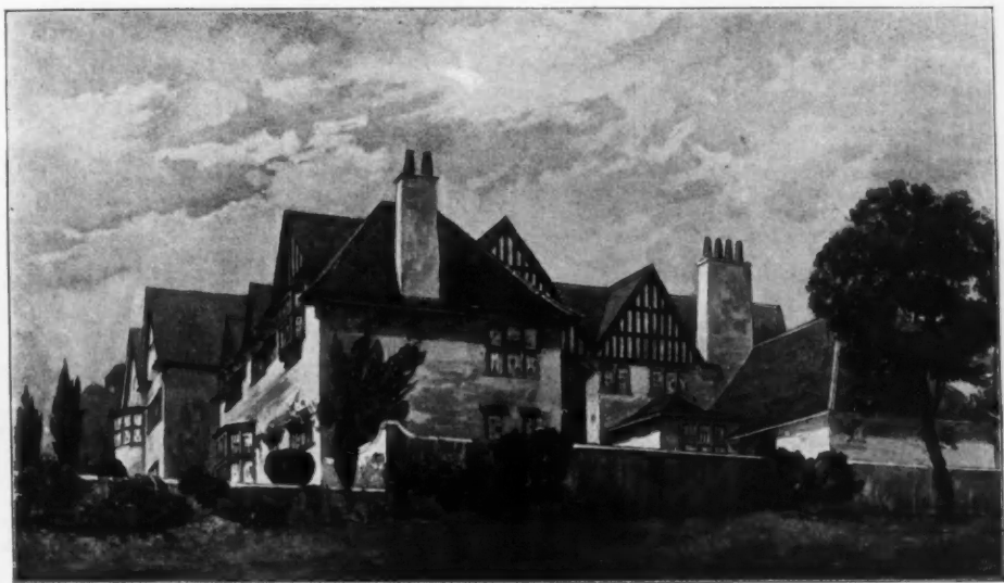
1829. Braham, Perth , F. W. BEDFORD AND S. D. KITSON, Architects. (For plan, see p. 142).
