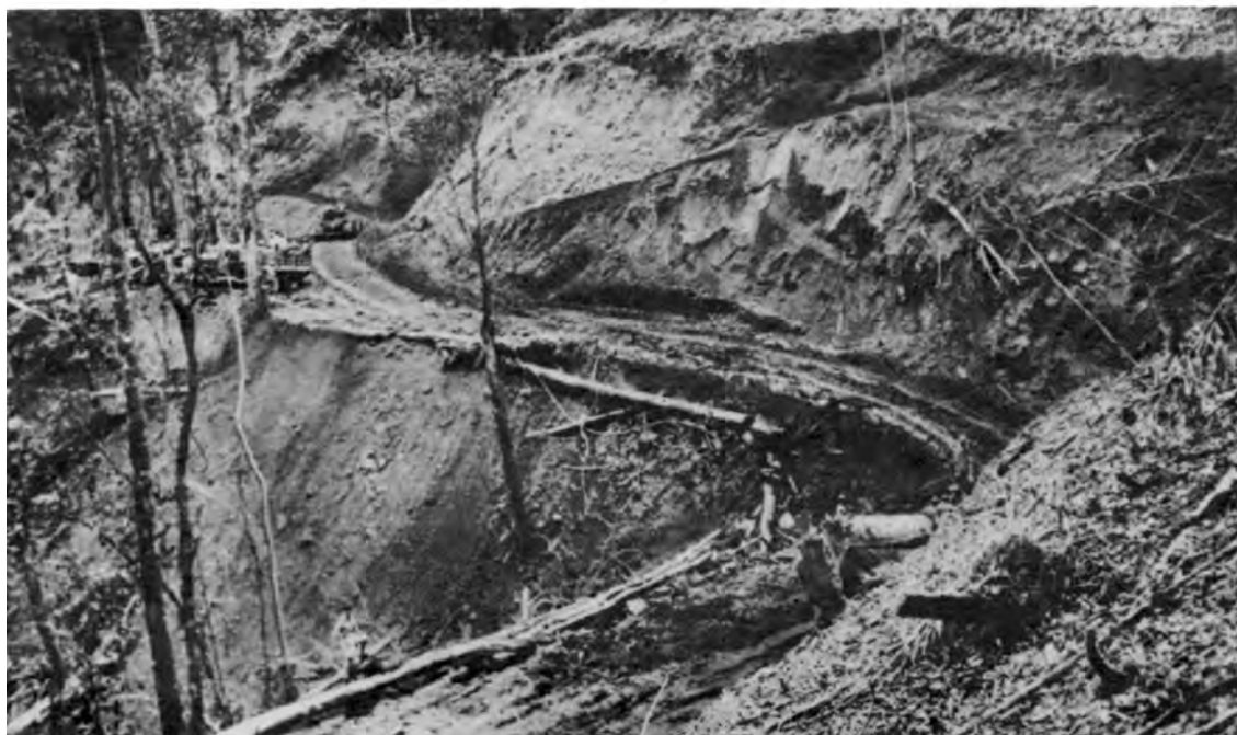
CONSTRUCTION WORK ON THE LEDO ROAD, 1943. U.S. Army Engineers supervise the building of a bridge by natives, above. Below, a curve on the road is cut into the hillside by bulldozers.
